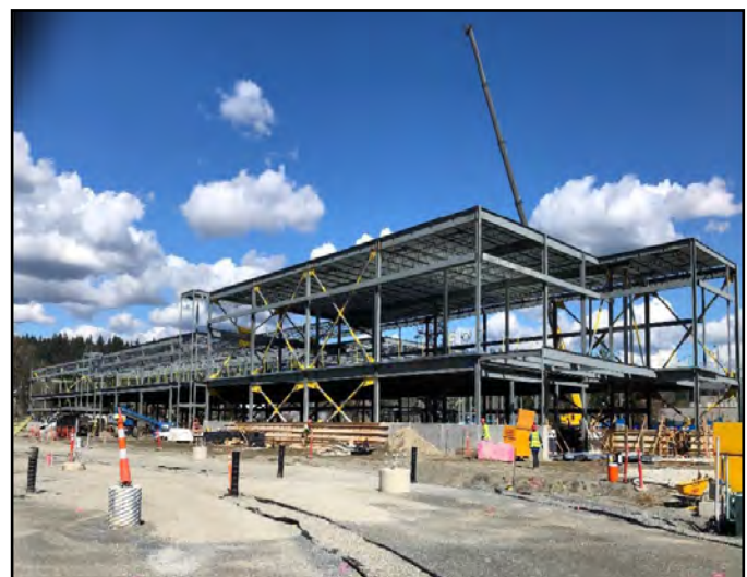
Structural Steel Erection at OMF East Building.
