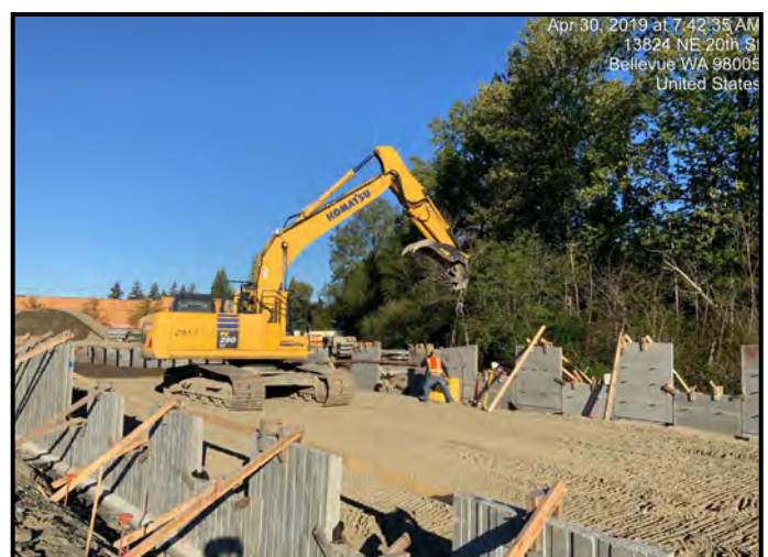
Work Area 2— MSE Wall Panel Set and Backfill
