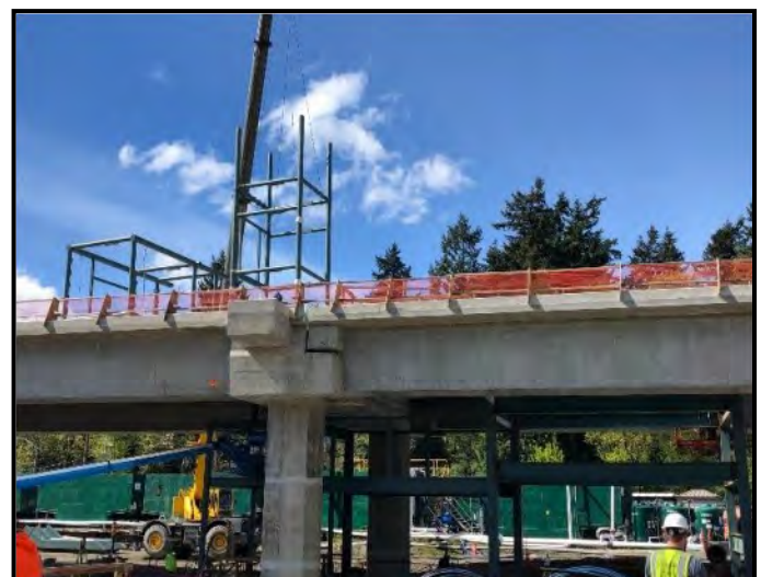
Progress on the station platform—placing structural steel.
