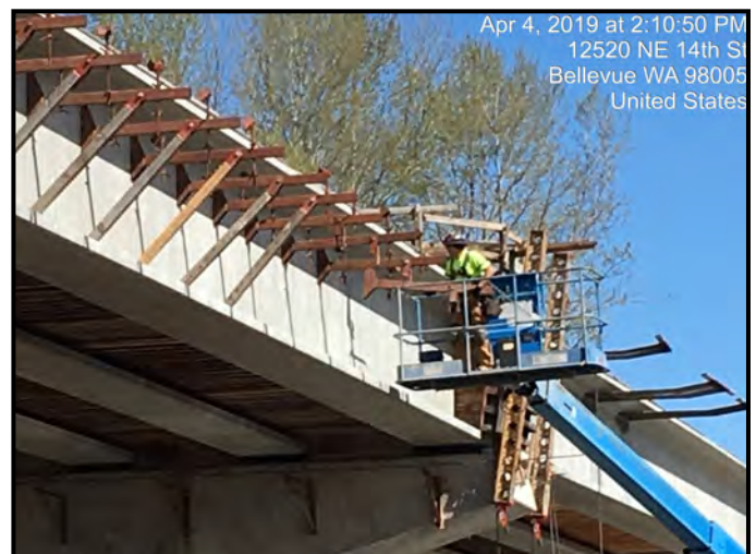
Installing the south side overhand brackets looking northeast.
