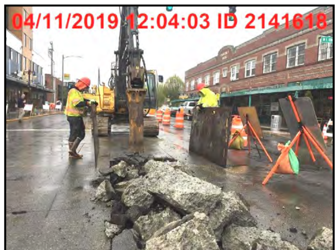
Sewer crew breaking roadway at intersection of 11th and MLK.
