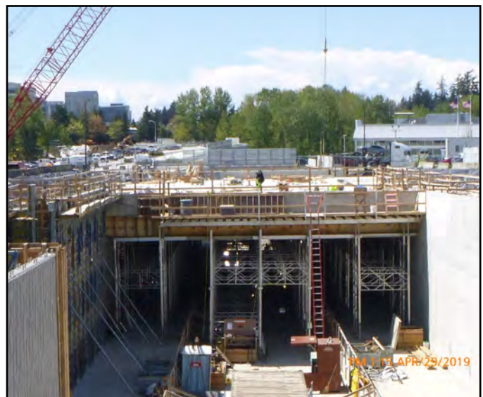
Strip out false work at 120th Station (Area 6)
