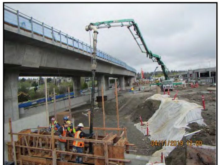
Crews placing concrete for north bridge abutment.
