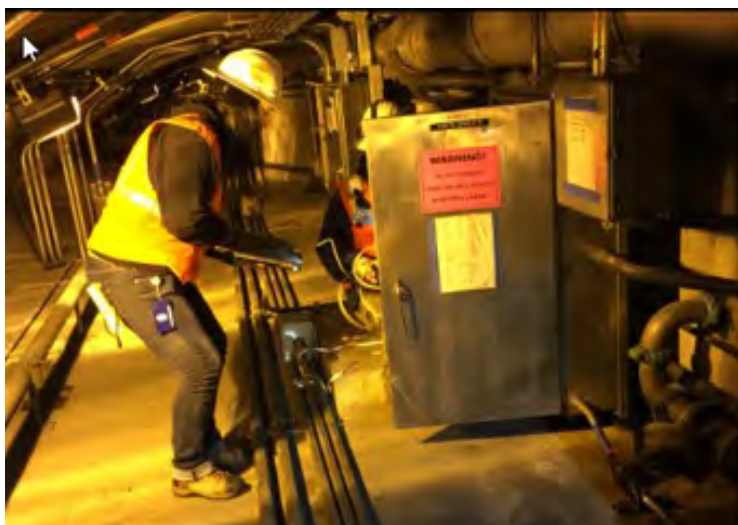
Crews verifying data connections for F/L/S System interface, Mt. Baker Tunnel plenum
