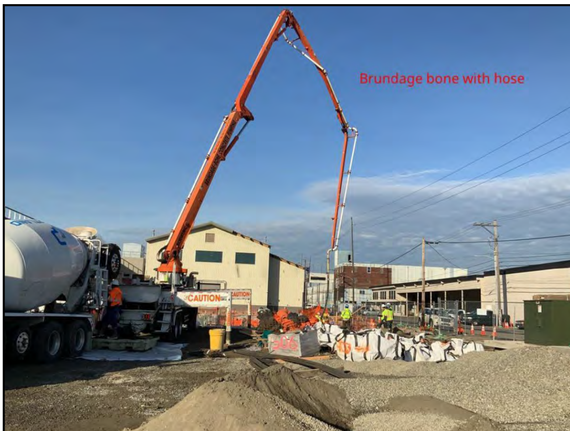
OMF-Mason subcontractor pumping concrete to elevator, service pit and truing pit slabs.
