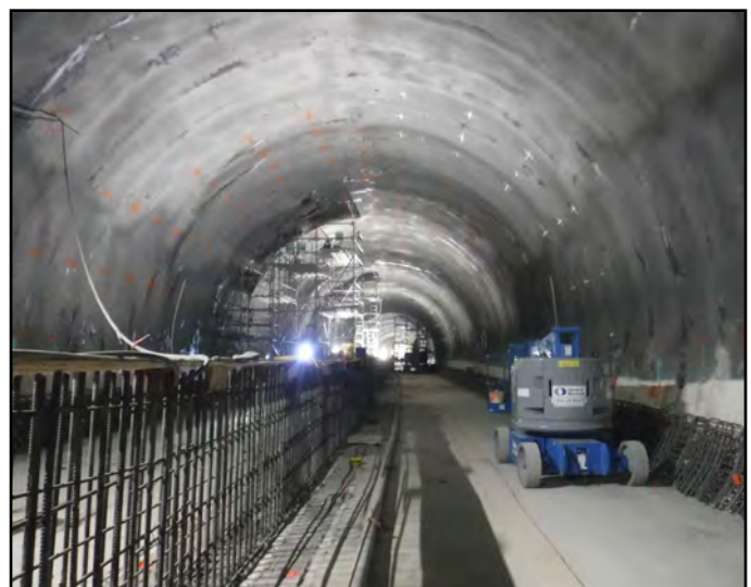
Moving Scaffold to grind and patch crown.
