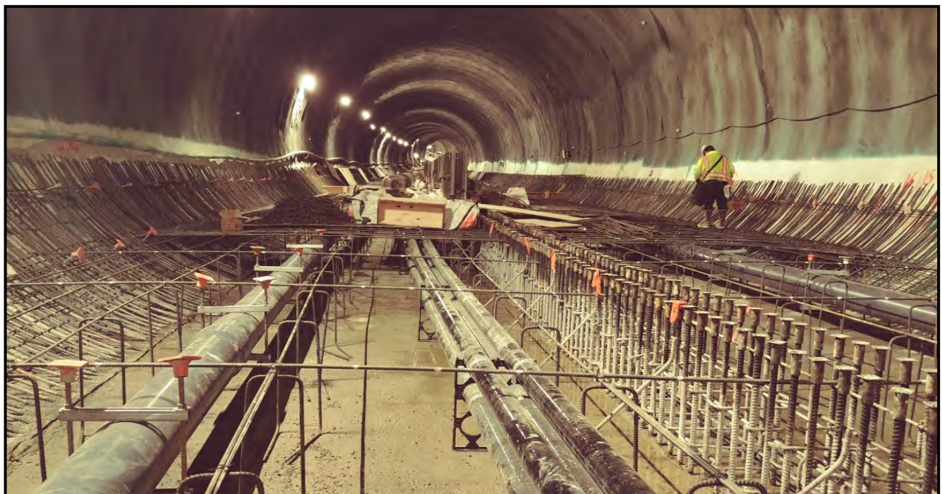
E330 Downtown Bellevue to Spring District : Rebar work and Conduits on the tunnel floors.
