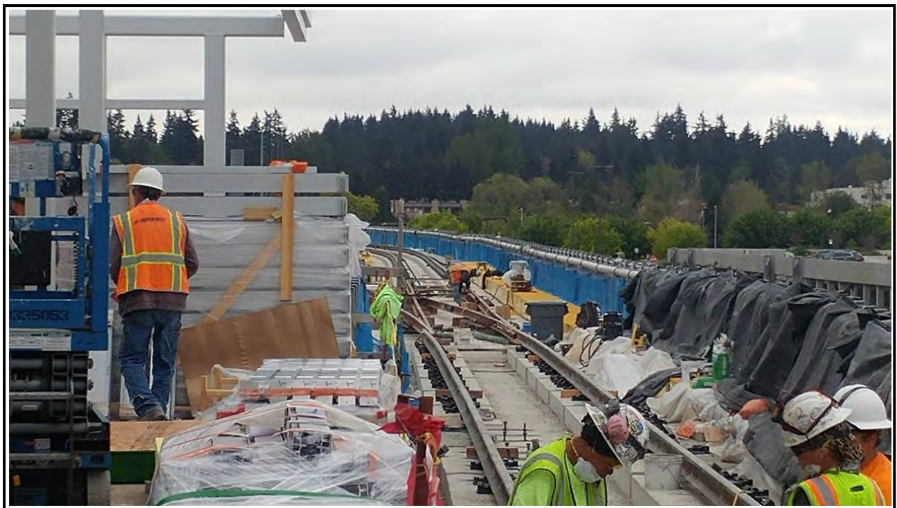
N180 - Crews installing special trackwork at north end of elevated guideway at Northgate.
