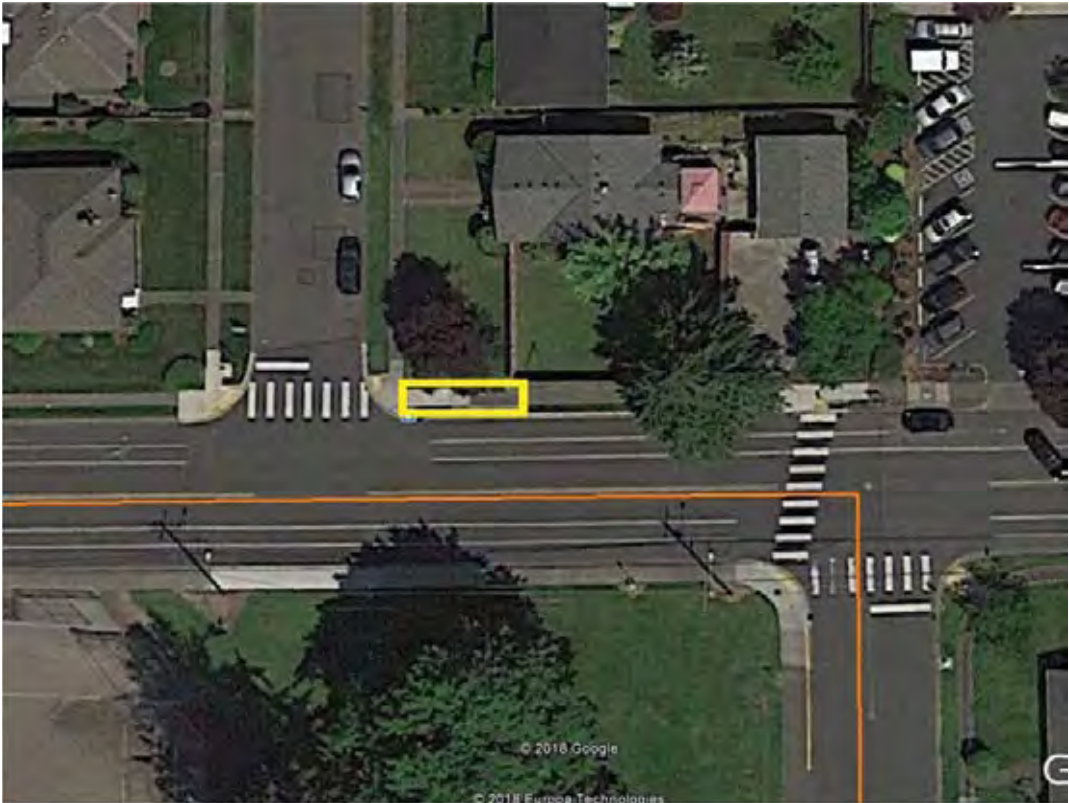
Bus Shelter Site 3: Westbound 17th Street SE, J Street SE
