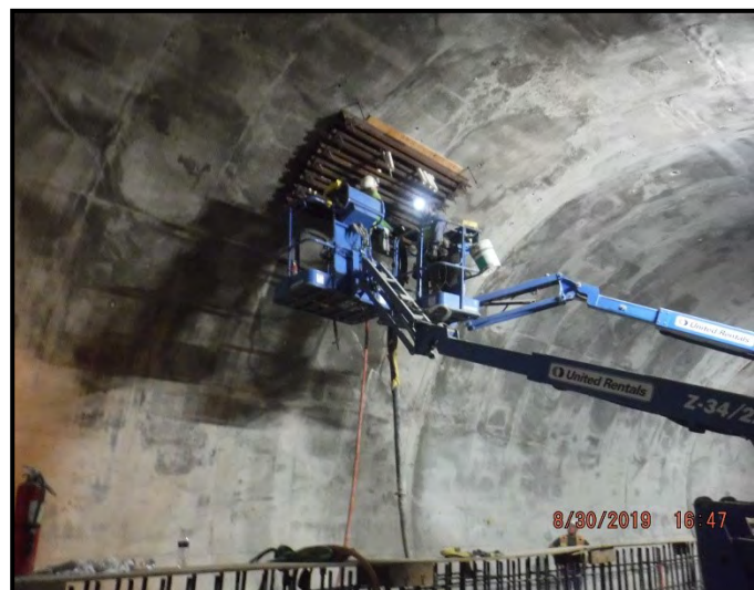
Repair crown final lining by placing concrete .
