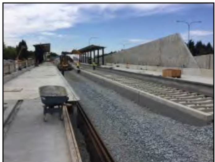
Overlake Village Station—Placing Concrete Ties
