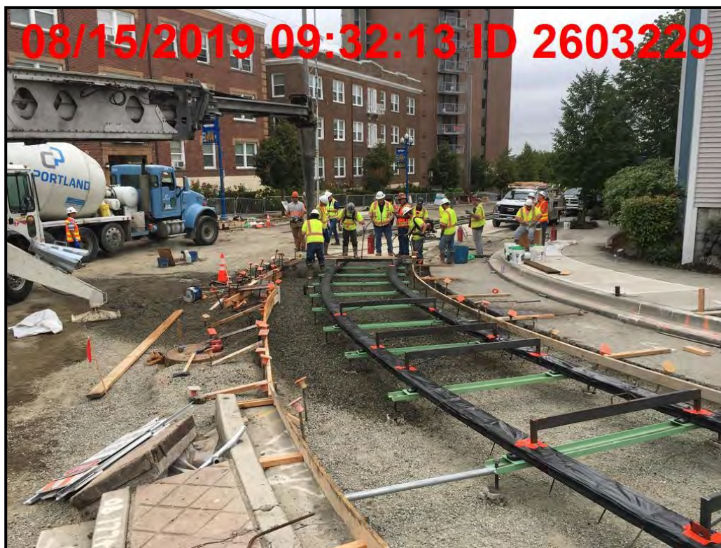
Placing Concrete for Track Slab south of Station
