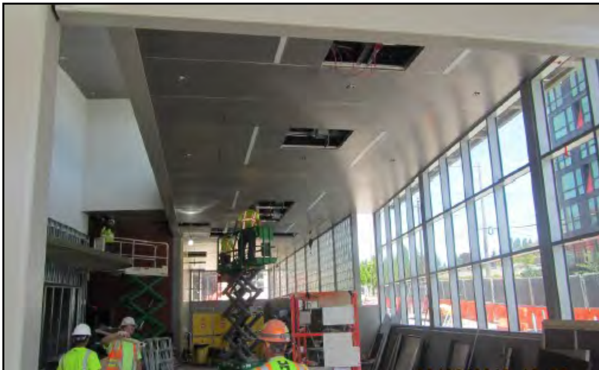
N140 – Sprinkler Installation.
