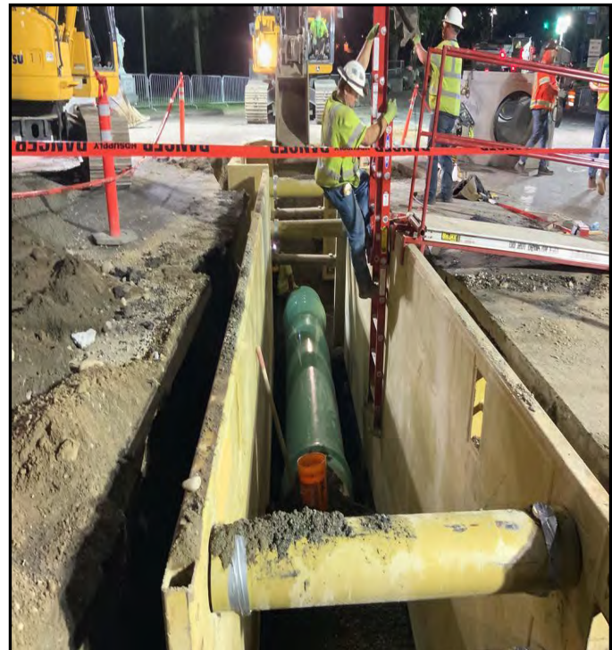
Night crew installing storm drainage
