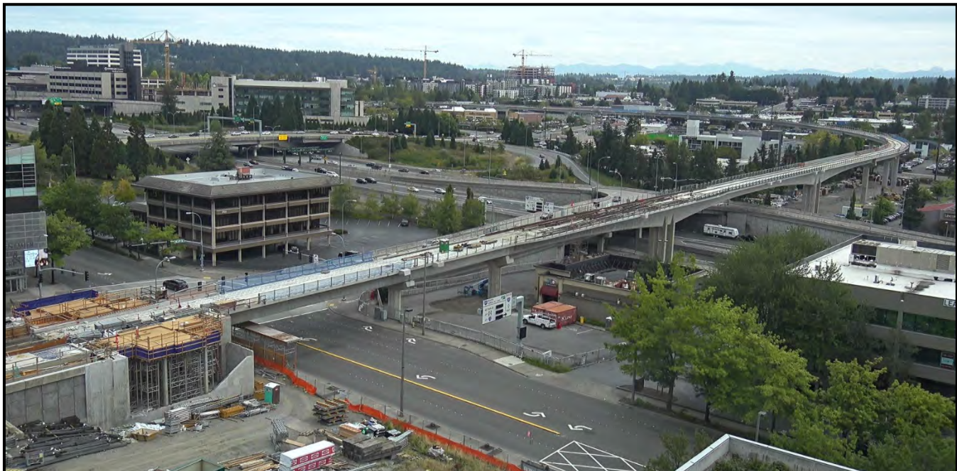
E335 Downtown Bellevue to Spring District: Bridge spanning over Highway I-405 along NE 6th Street on August 31, 2019.
