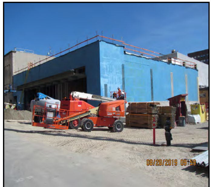
U District Station – Weather Air Barrier at North Headhouse
