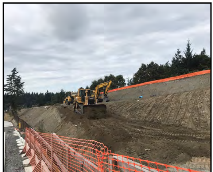
Work Area 6—Regrading the slope.
