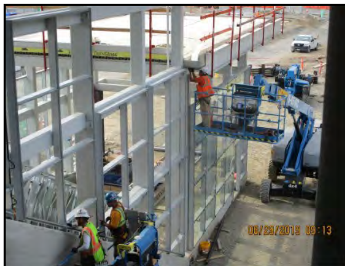
Installation of glass screen wall frames at station entrance.
