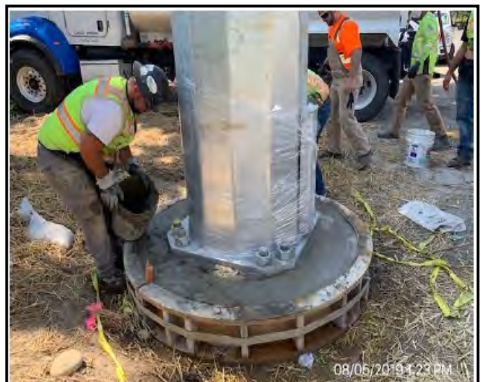
Seattle City Light transmission pole foundation.
