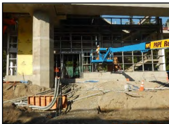
Curtain wall (glass wall) work at station
