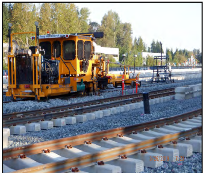
Track-work, Ballast Adjustment
