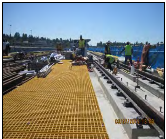
Crews working on walkway in WA 7.2
