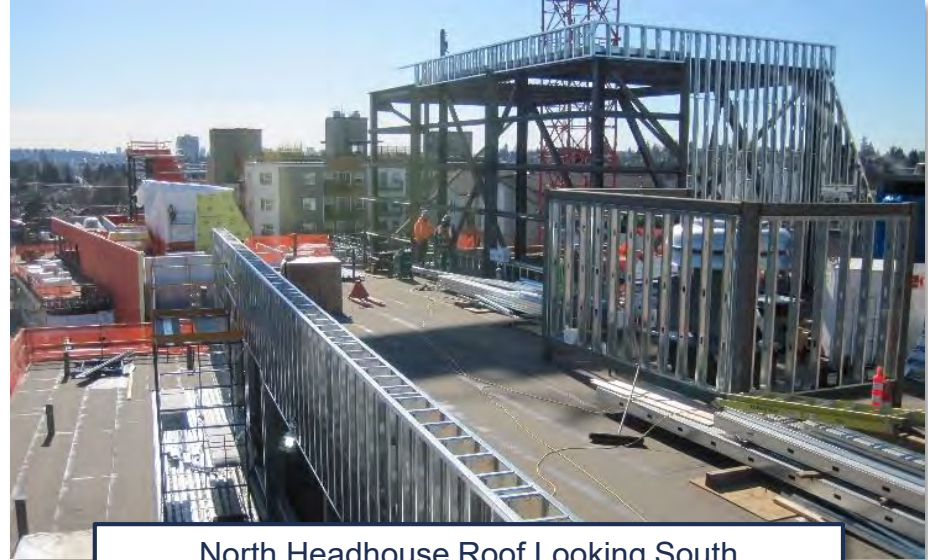
North Headhouse Roof Looking South
