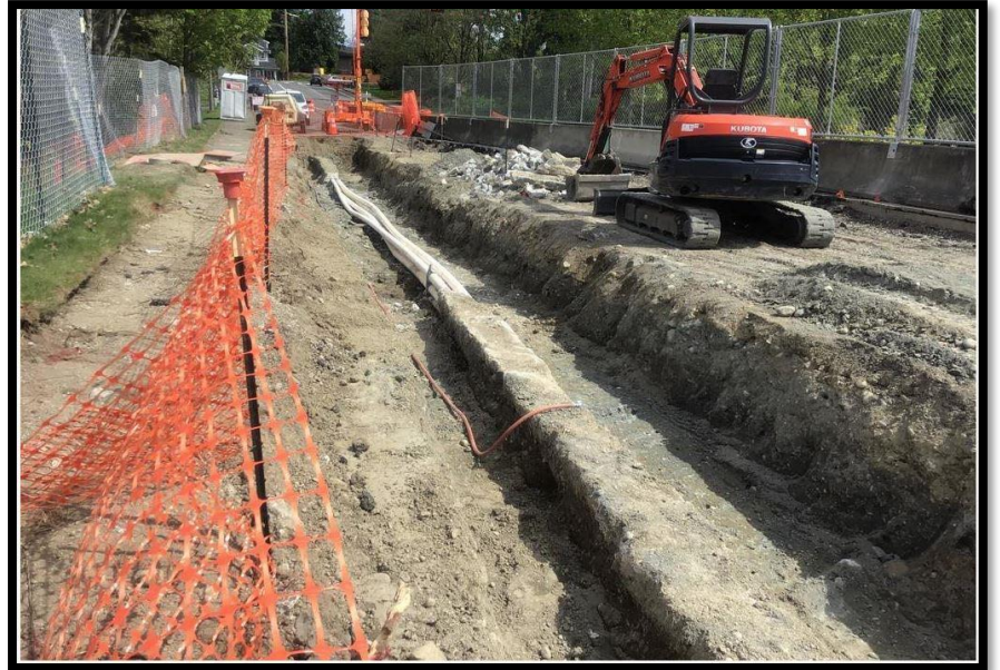
Third-party utility work, relocation of existing duct bank 60th Street.
