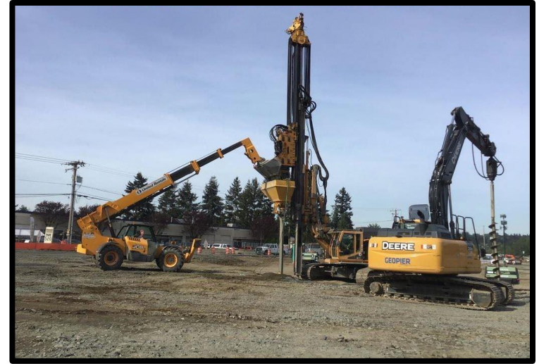
Installation of geo pier at the future Southeast Redmond Station and Garage
