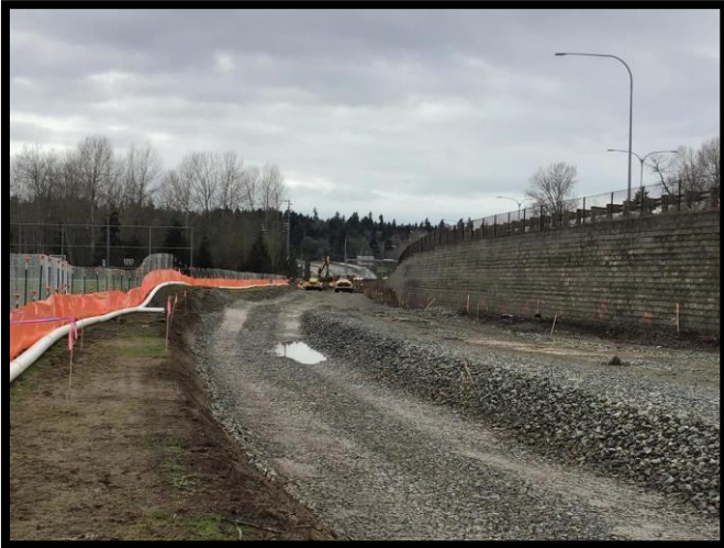
Access road along Marymoor Park, facing west on SR 520 eastbound.
