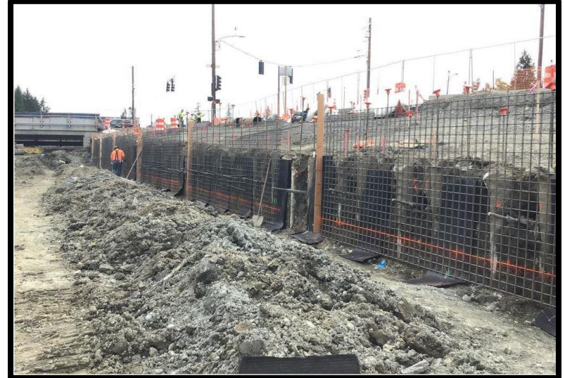
Soil nail wall install mesh and rebar near NE 51st Street
