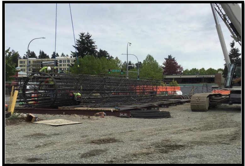
Fabrication and assembly of shaft rebar cage at Downtown Redmond Station
