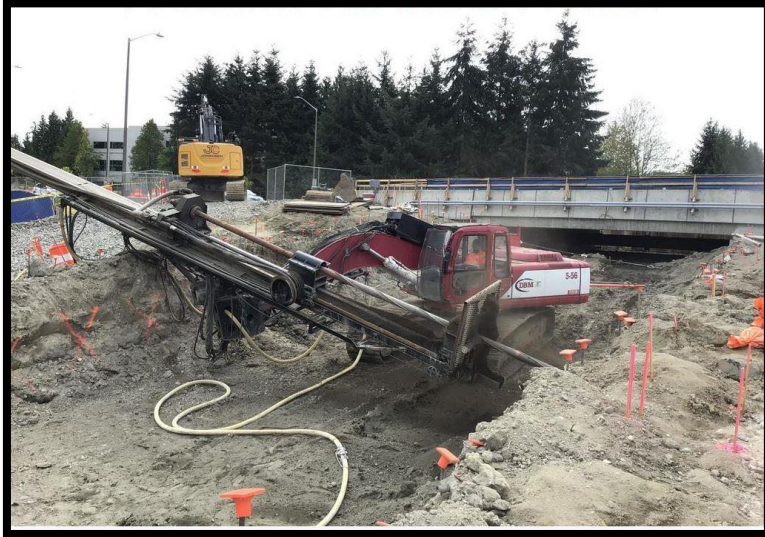
Soil nail wall work near NE 51st Street undercrossing 51st Street undercrossing
