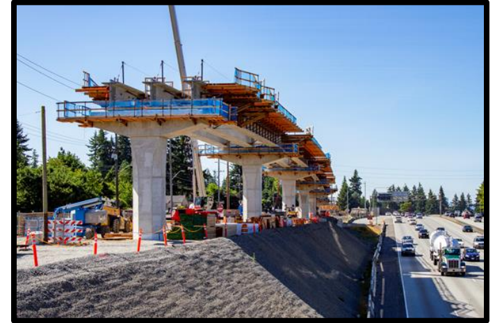
Bridge Adjacent to I-5 Near NE 130 th Street and 5 th Avenue NE in Seattle
