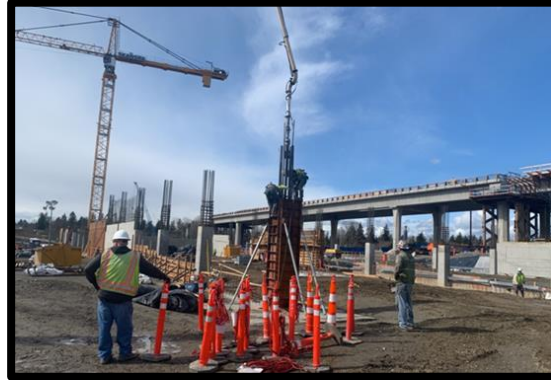
Concrete Placement for Columns at Lynnwood Station Garage
