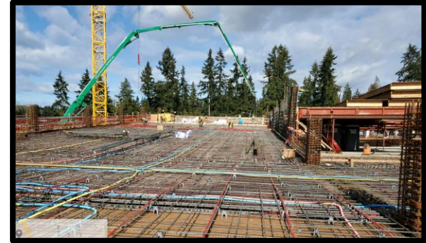
Concrete Deck Placement at Shoreline 148th Station Garage
