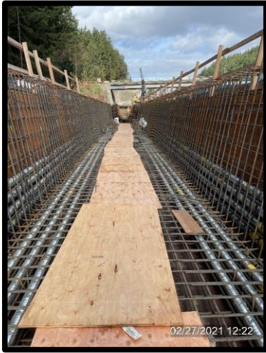
Rebar Placed for I-5 Overcrossing Stem Walls
