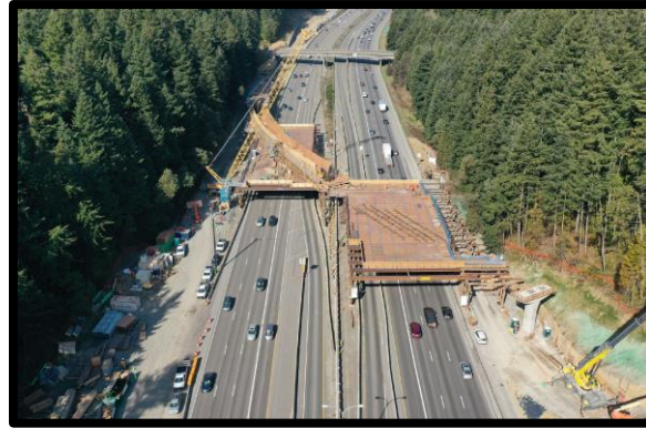
Formwork Placement in Progress Across I-5
