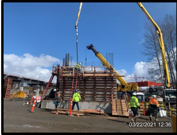
Placing Concrete for a Shear Wall at the Lynnwood Station Garage
