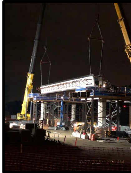
Setting Girders at Shoreline South / 148 th Station
