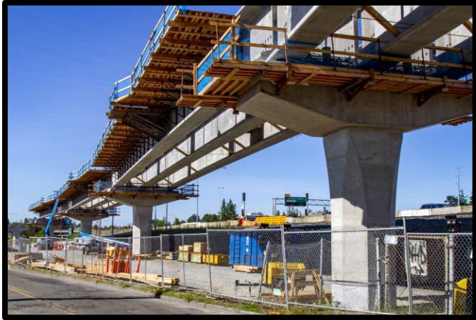
Guideway North of Northgate Station and East of I-5 at N 115 th Street
