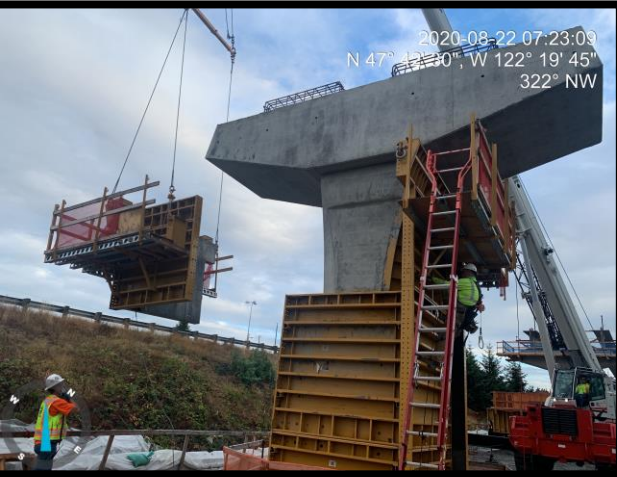
Removing Steel Forms for Column and Bent Cap in Seattle at 112th St and 1st Avenue East of I-5
