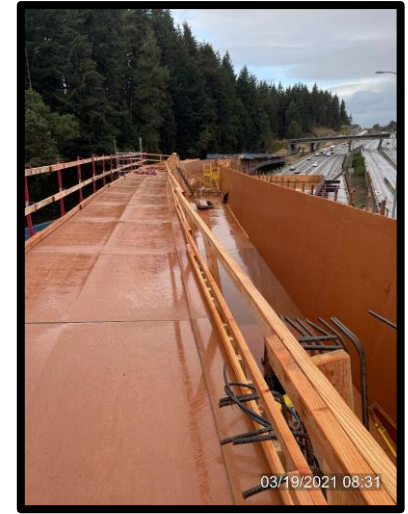
Bridge Overhang Decking over I-5 Facing North
