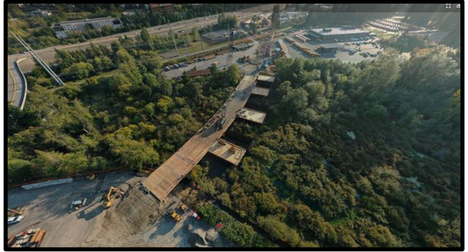
Scriber Creek Trestle in Lynwood
