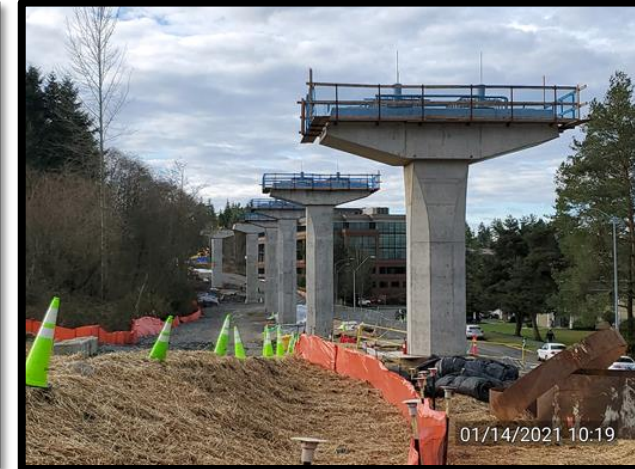
Columns West of I-5 Looking South in Mountlake Terrace at St Albion Way
