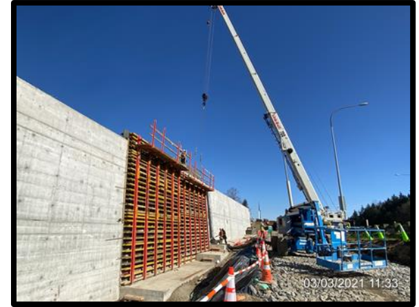
Placing Rebar for Wall in Mountlake Terrace
