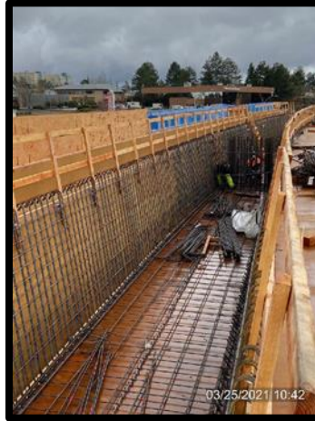
Placing Rebar for Longspan Bridge over I- 5 in Mountlake Terrace
