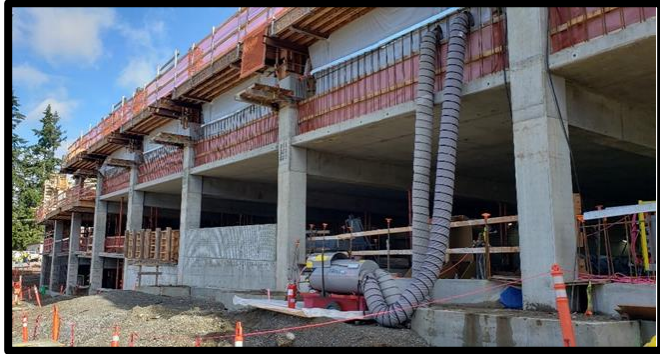
Progress on Fourth Level of Shoreline South / 148th Parking Garage
