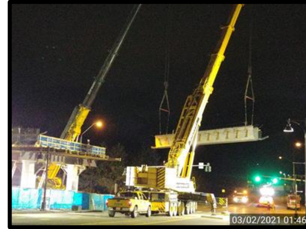
Girder Installation of 236 th St SW East of I-5 at Mountlake Terrace Station
