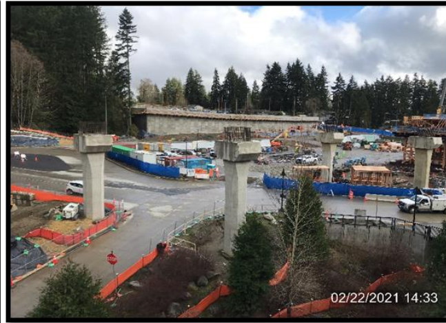
Guideway Columns at Mountlake Terrace Station site
