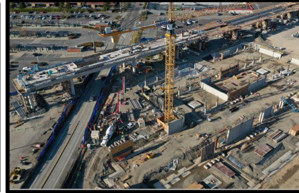
Aerial View of Lynnwood Station and Parking Garage
