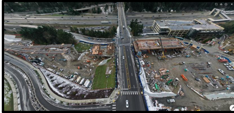
Aerial View of the Mountlake Terrace Station site
