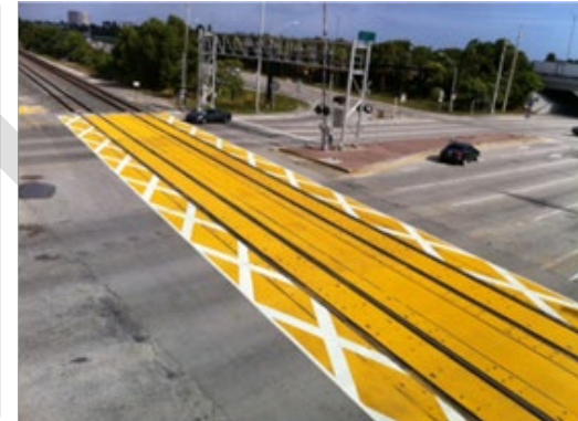
Figure (left): Sample DO NOT STOP ON TRACKS signage Figure (right): Sample dynamic envelope pavement markings
