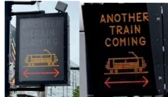
Figure: Example Another Train Coming signs
