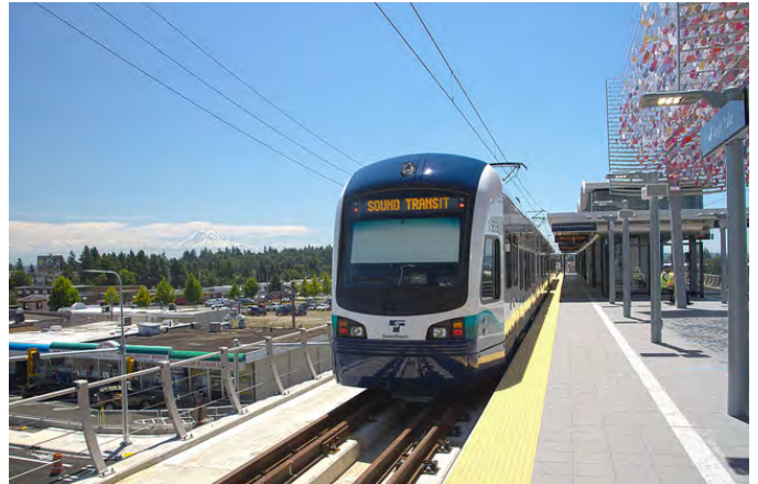
An example of direct fixation track at Angle Lake Station, SeaTac
