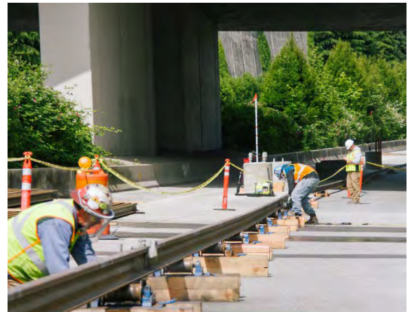
Crews grind and inspect welds along an assembly line
