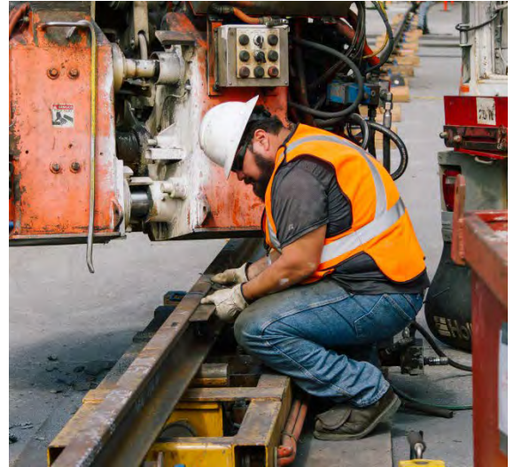
A worker aligns rails to be ‘flash butt’ welded by machine
