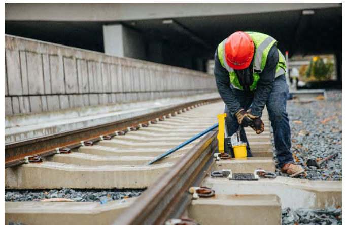
An example of ballasted track on Mercer Island.
