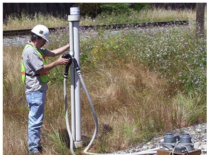
Example of noise and vibration monitoring equipment
