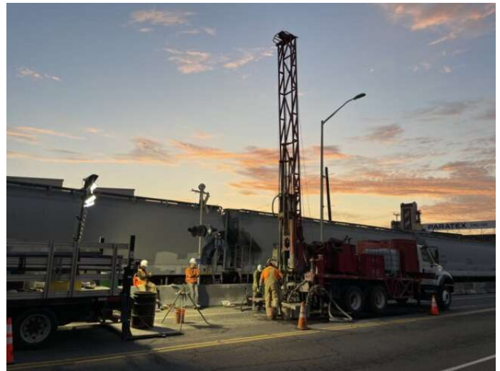
Example of geotechnical drilling equipment
