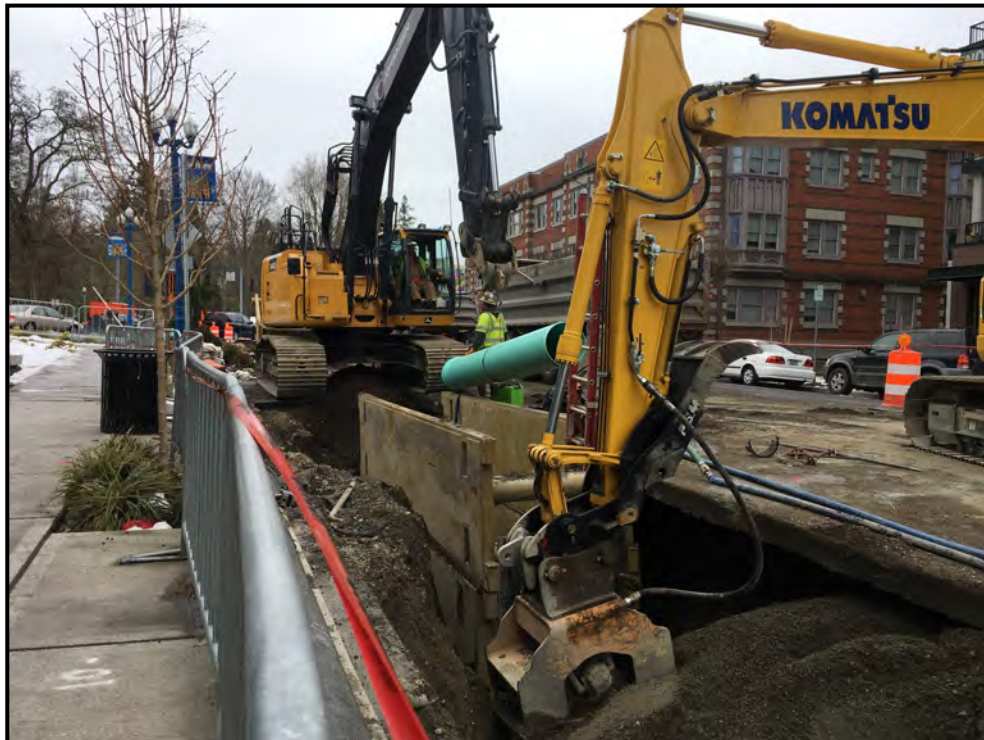
Sewer pipeline construction in 1st Street
