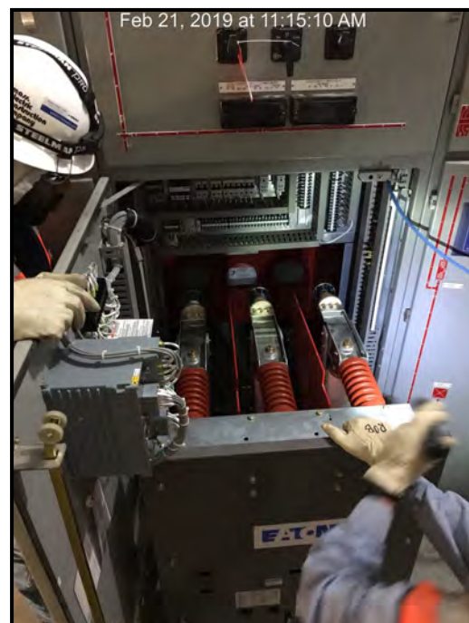
Installation of Breaker to the Racked Position of MVSS at Roosevelt Station, 02/21/2019.
