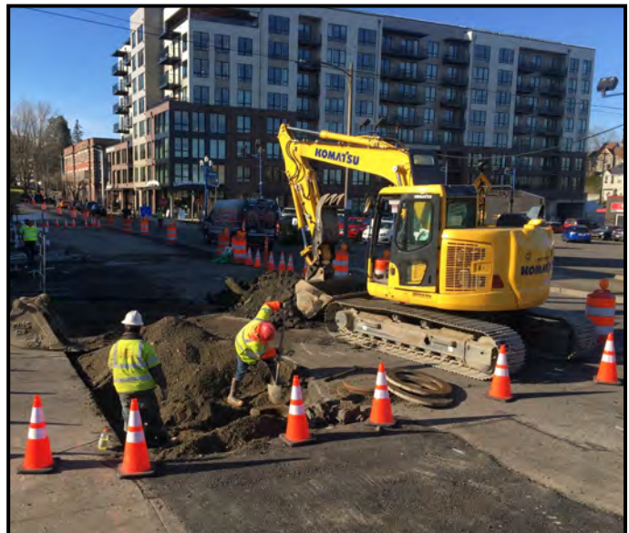
Excavating driveway and rebuilding manhole at Thriftway Market.
