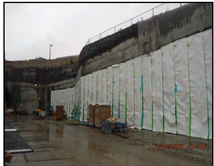
Installed waterproofing at South Portal Cut and Cover.
