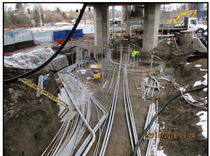
Electrical conduit layout at South Ancillary Room below the main station area.
