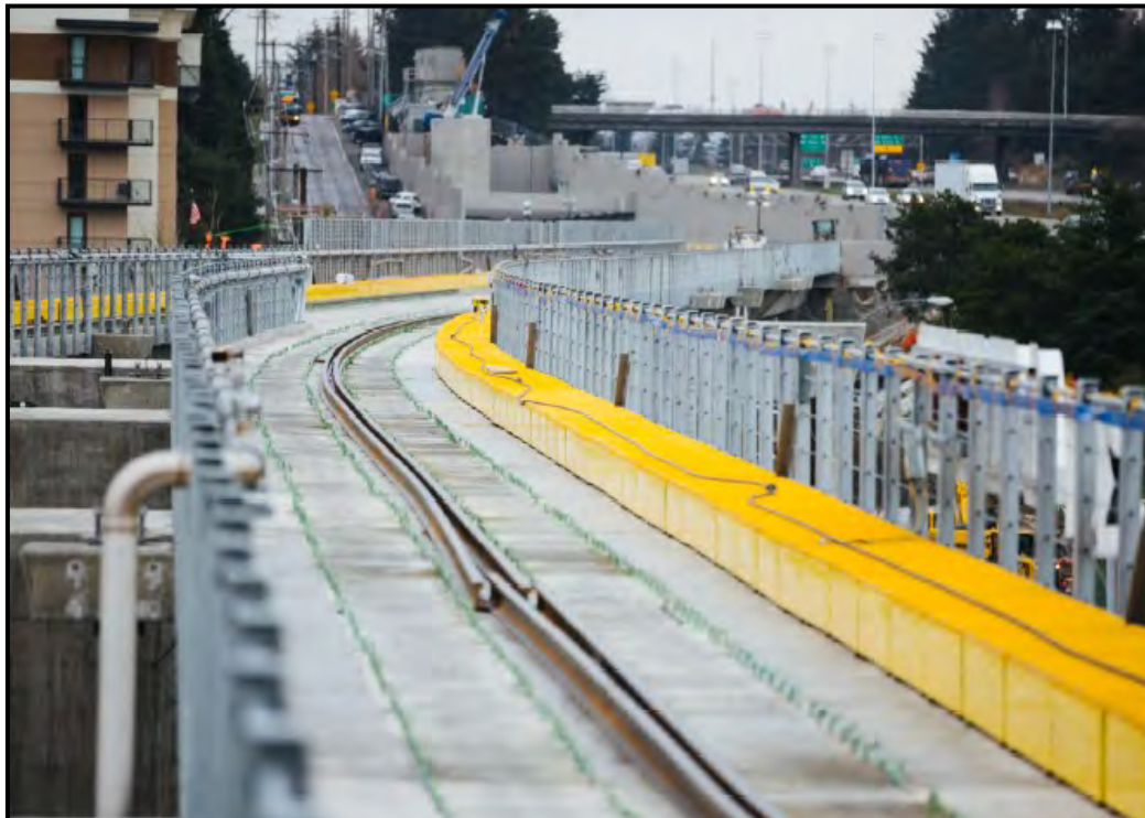
N180 - Crews completed pulling rail onto the elevated deck south of Maple Leaf Portal.
