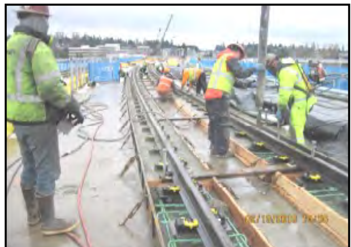
Placement of Direct Fixation Trackwork on the elevated deck at Northgate.
