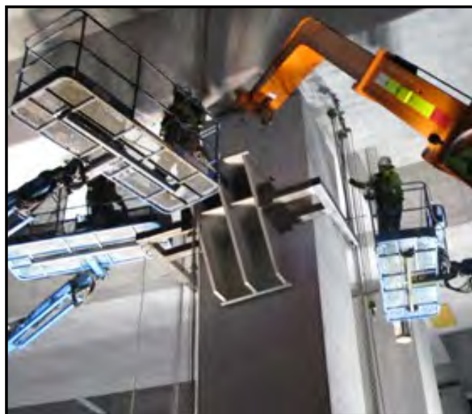
Installation of seismic restrainer bracket, D2 approach structure (West Segment)
