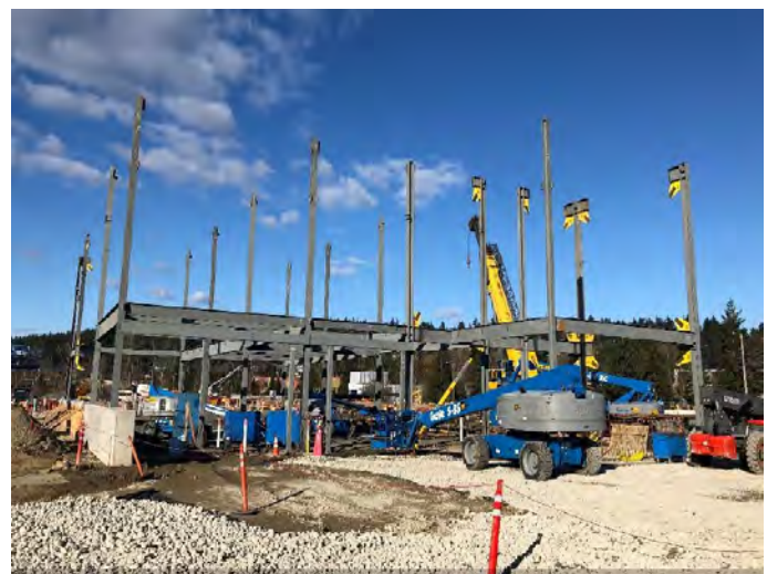
Structural Steel Erection at OMF East Building.
