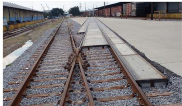
Typical Crossover Tracks: Allowing trains to move from one trackway to another.
