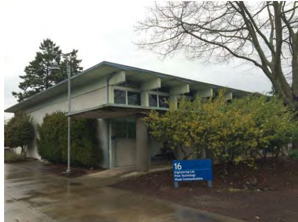
Southwest corner, west wing 2014
