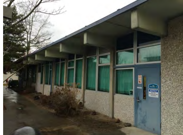
South elevation, view to the northwest 2014
