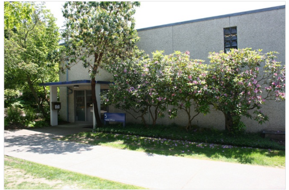
Highline College Building 5, Northwest Corner
