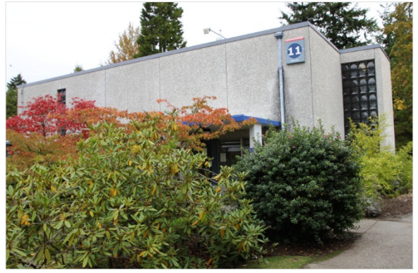
Highline College Building 11, Southwest Corner
