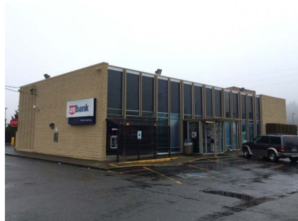
US Bank, Southwest Corner
