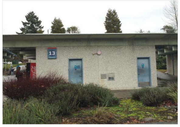
Highline College Building 13, West Elevation
