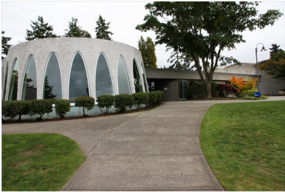
Highline College Building 4, West Elevation
