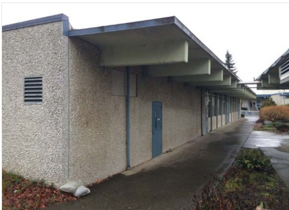
Highline College Building 12, Northeast Elevation
