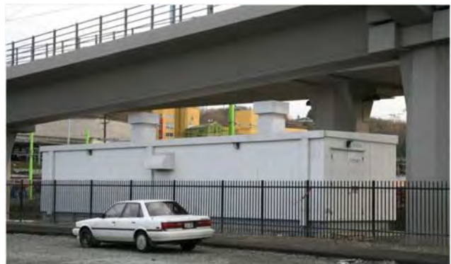
EXHIBIT 2-6 Traction Power Substation
