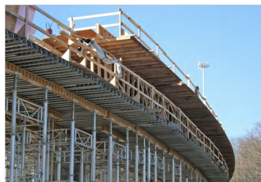
Construction of Elevated Guideway Showing False-Work
