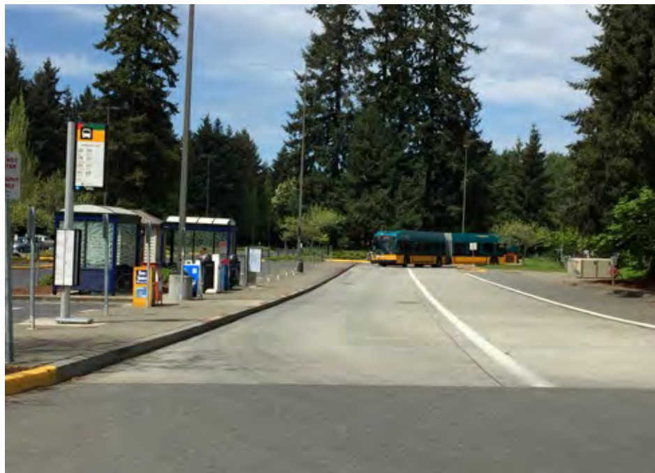
Existing bus service facilities
