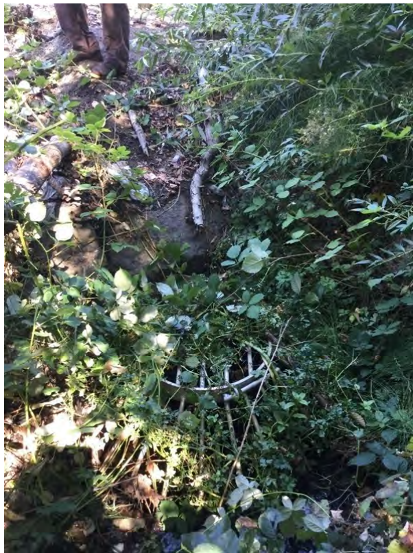
Photo 13. Overflow culvert at end of STU-2 and STU-3
