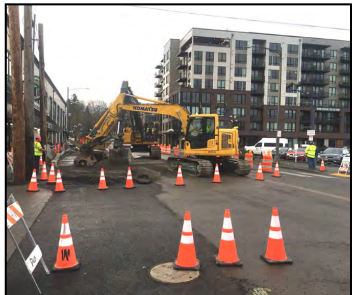
Restoring trench line south of Thriftway Market driveway.
