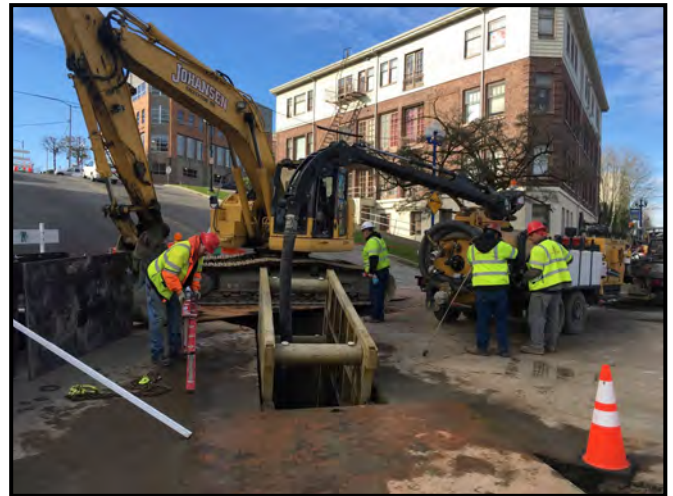
Vacuum extracting sub grade for shoring box installation.
