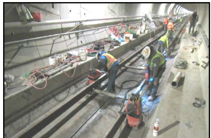
SWI—Continuing their drilling for the DF stirrup bar placement in the invert of the SB tunnel of WA.5.
