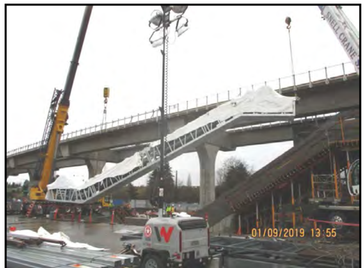
Placing Escalator at Northgate Station.
