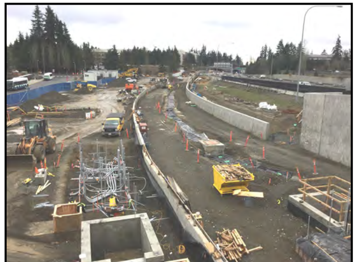
RTS (L2 garage looking west) - Track approach, electrical room and circulation tower foundation.
