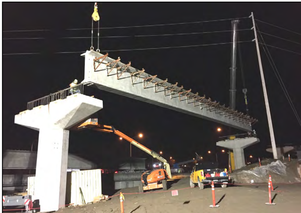
E360 SR520 to Redmond Technology Station: Span 16 Girder erection at the sweeper site along SR 520
