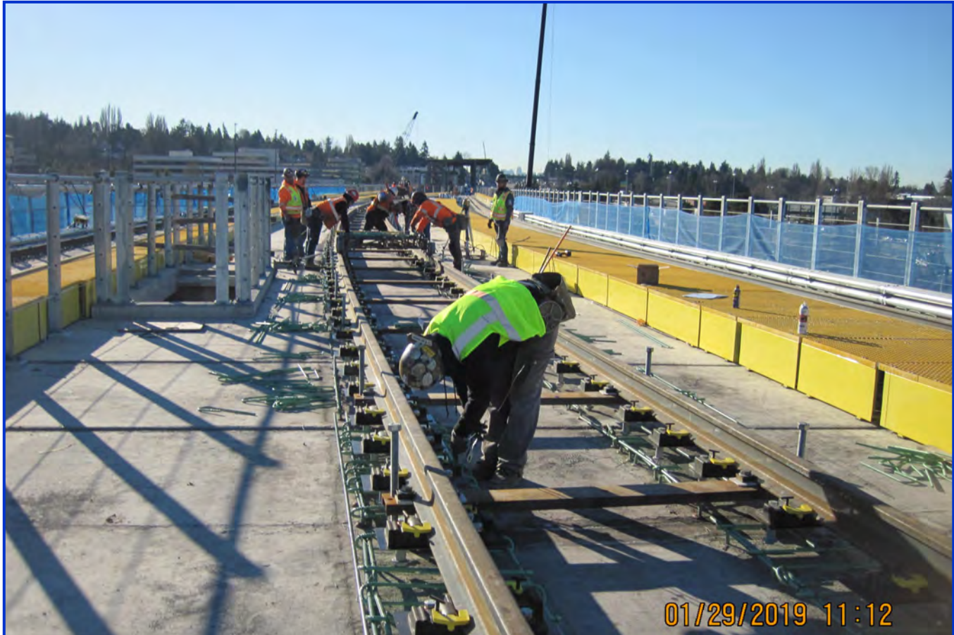
Crew constructing skeleton track for the pocket track of Northgate Link Ext.
