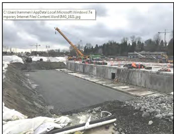
North Vault East base pad fine grade.
