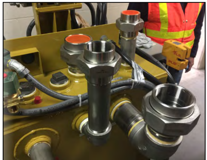
Inspecting MI Tunnel back-up generator fuel piping
