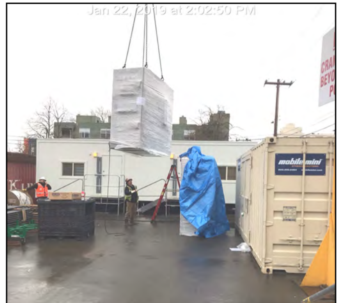
Offloading MVSS Switchgear with Tower Crane at Roosevelt Station, 01/22/2019.
