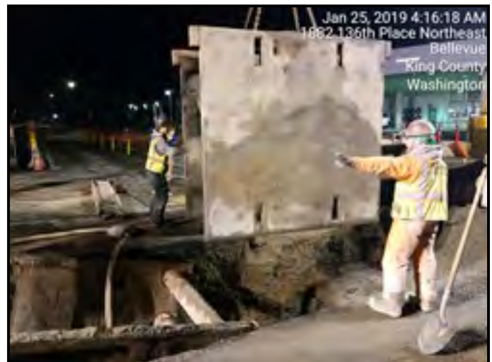
Placing trench box into open trench facing south.
