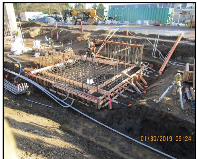
Elevator Pit rebar at Wilburton Station (Area 4)
