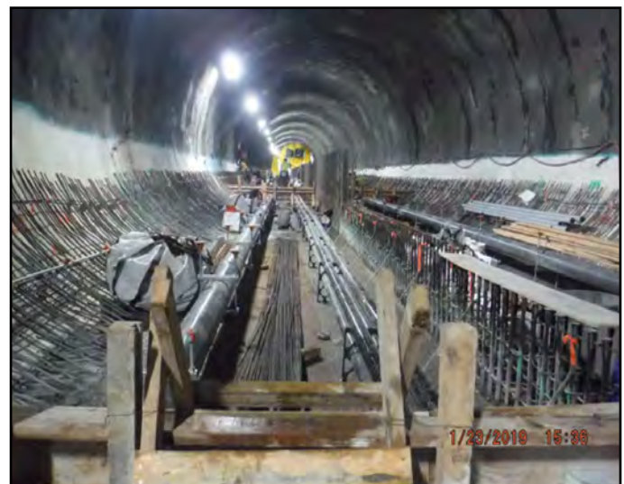
Rebar, conduit, and drain pipe installation.
