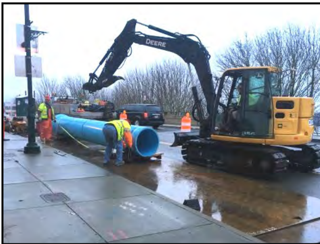
Crew preparing 30 inch casing for installation.
