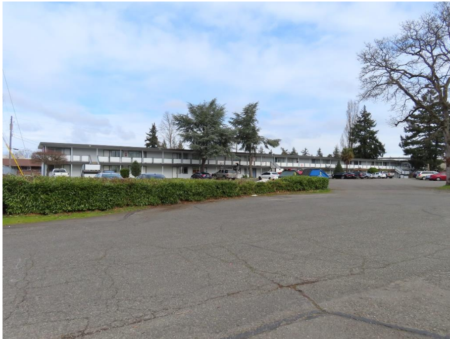
Figure 8-19 4801 115th Street Court SW, view northwest
