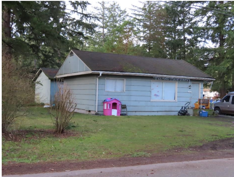
Figure 8-41 5508 Boston Avenue SW, view west
