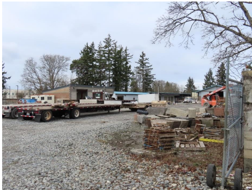
Figure 8-17 4610 113th Street SW, view northwest
