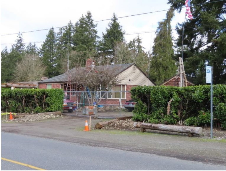
Figure 8-35 4911 McChord Drive Street SW, view northwest
