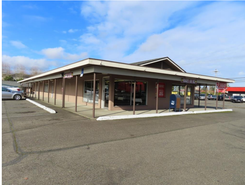
Figure 8-5 11202 – 11208 Bridgeport Way SW, view northwest
