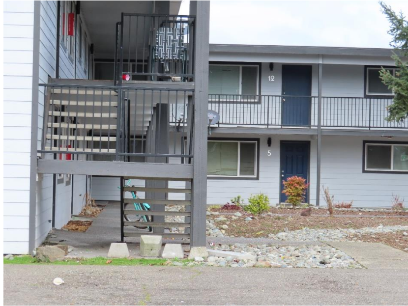
Figure 8-23 4901 115th Street Court SW, view north
