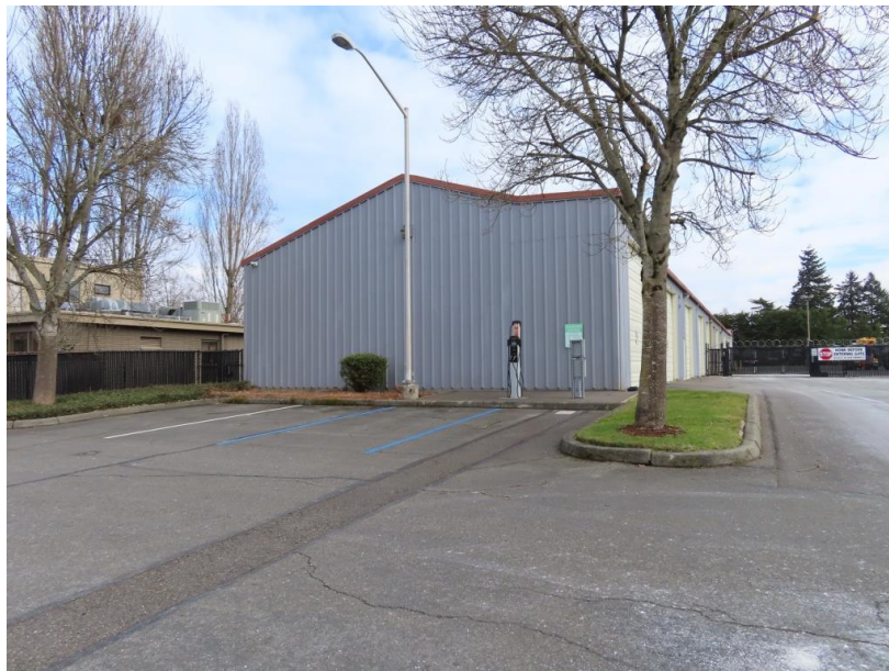
Figure 8-24 11509 Bridgeport Way SW, view east
