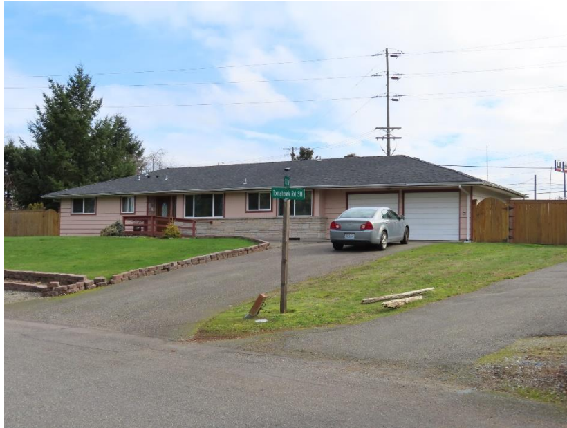
Figure 8-29 11811 Tomahawk Road SW, view northeast
