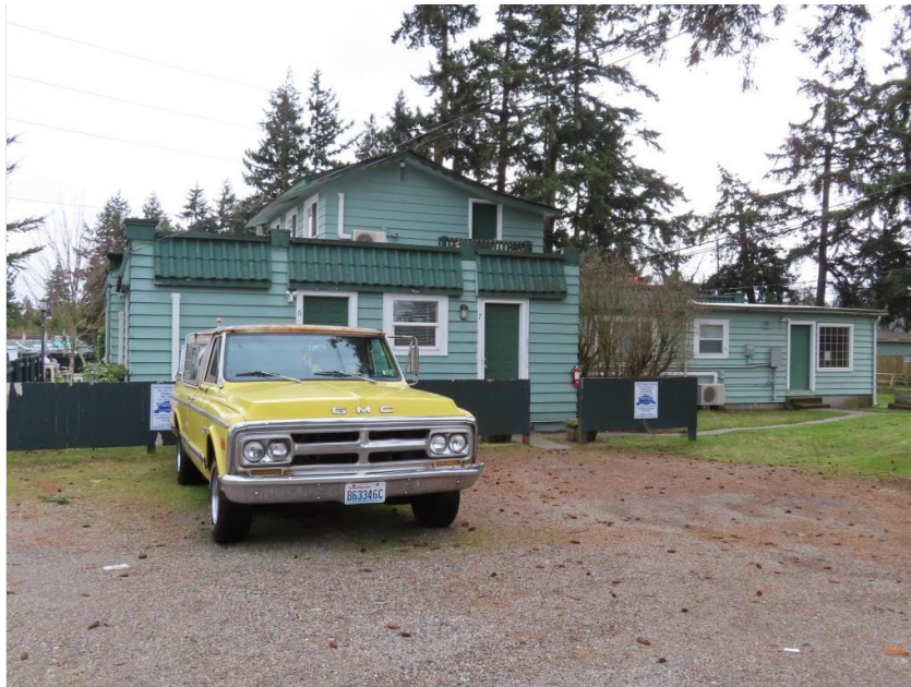
Figure 8-8 4400 Lakeview Avenue SW, view southeast
