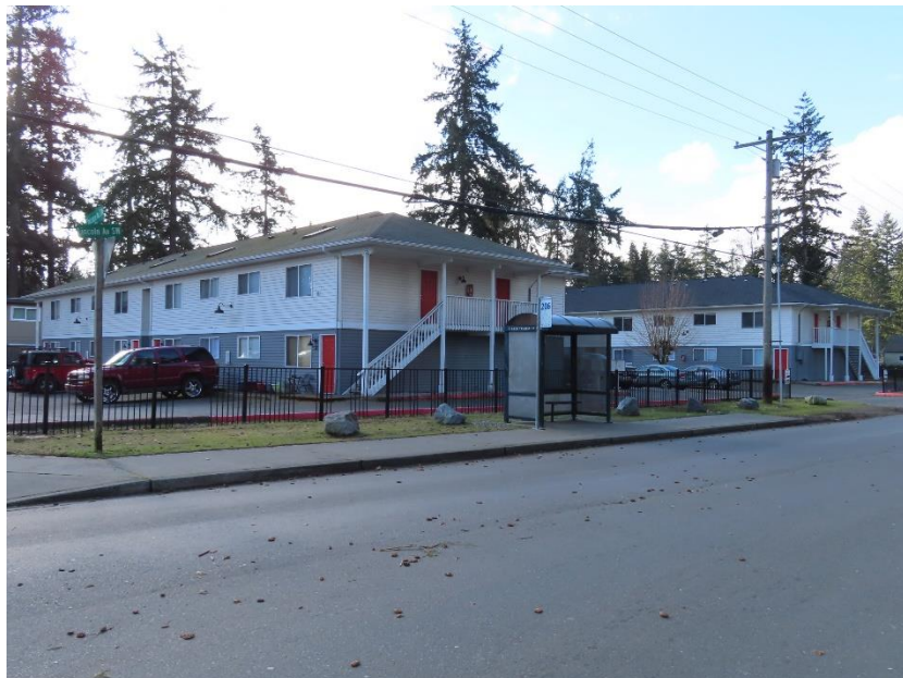
Figure 8-38 12809 Lincoln Avenue SW, view southwest
