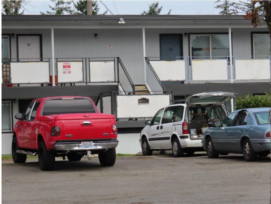
Figure 8-20 4801 115th Street Court SW, view north
