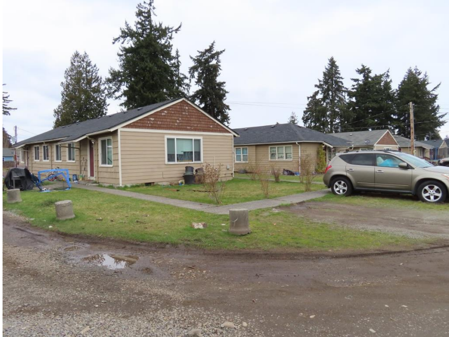
Figure 8-13 11216 – 11230 Kline Street SW, view northwest
