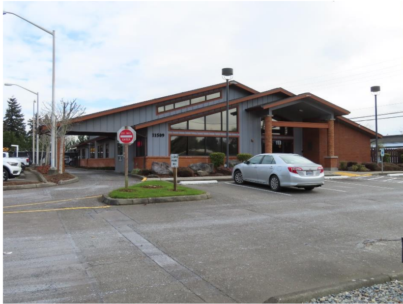
Figure 8-25 11509 Bridgeport Way SW, view northeast
