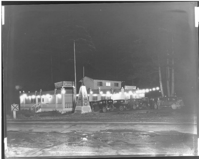
Figure 8-10 4400 Lakeview Avenue SW, view southeast
