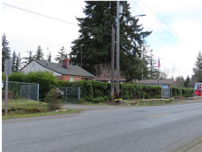
Figure 8-36 4911 McChord Drive SW, view northeast
