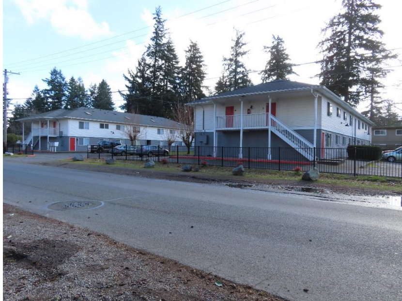
Figure 8-37 12809 Lincoln Avenue SW, view southeast
