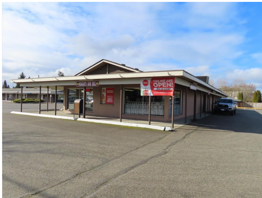
Figure 8-4 11202 – 11208 Bridgeport Way SW, view southwest
