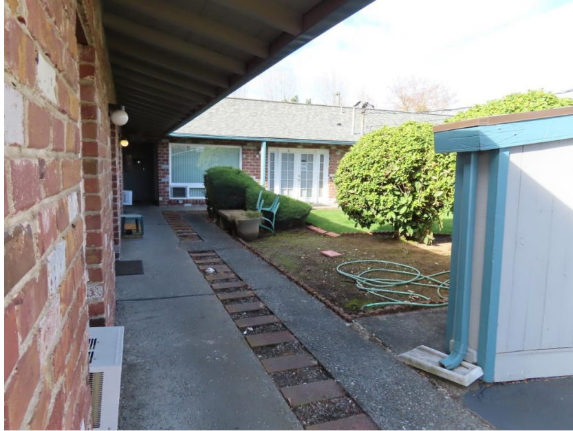
Figure 8-2 5202 112th Street SW, view northwest
