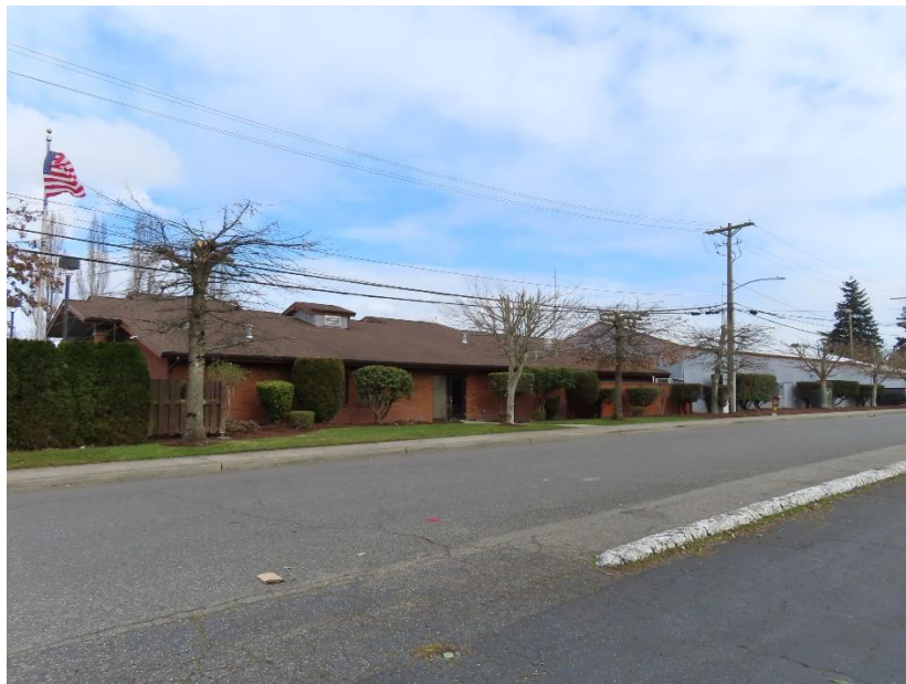
Figure 8-26 11509 Bridgeport Way SW, view east
