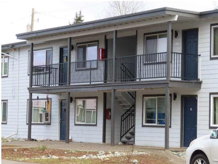
Figure 8-22 4815 115th Street Court, view northeast
