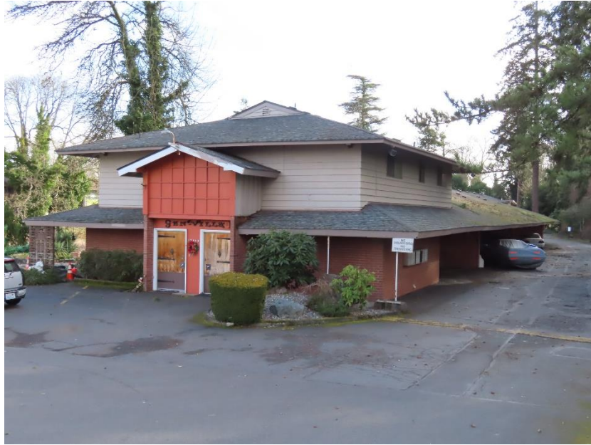
Figure 8-31 12413 Bridgeport Way SW, view east
