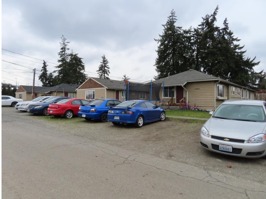
Figure 8-15 11216 - 11230 Kline Street SW, view southwest
