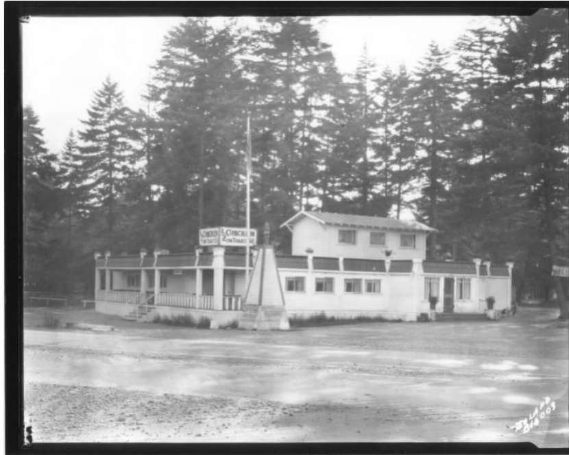
Figure 8-9 4400 Lakeview Avenue SW, view southeast
