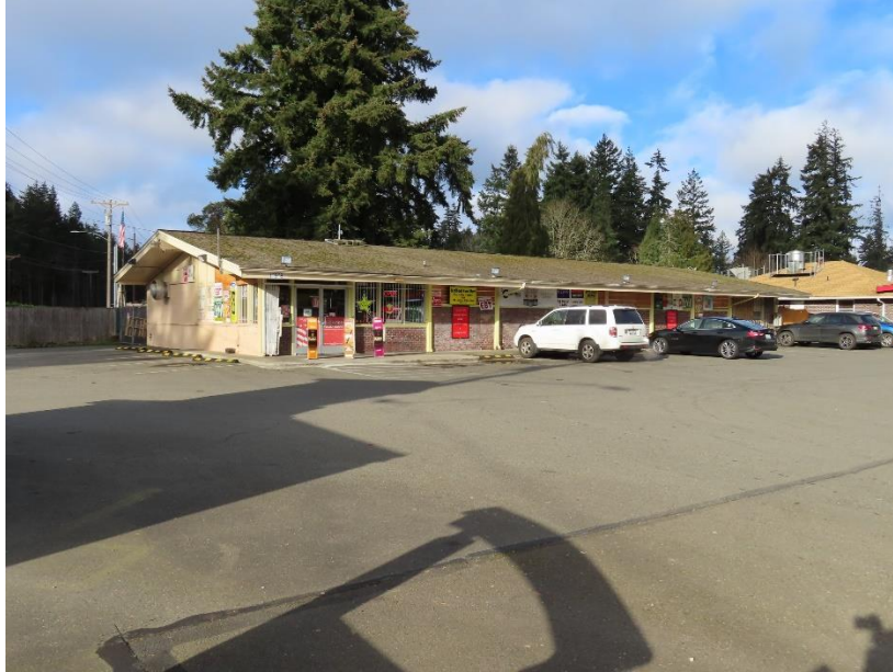
Figure 8-33 12928 Bridgeport Way SW, view northeast
