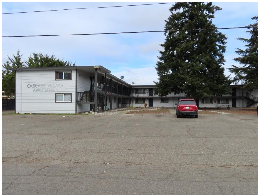
Figure 8-22 4901 115th Street Court SW, view north
