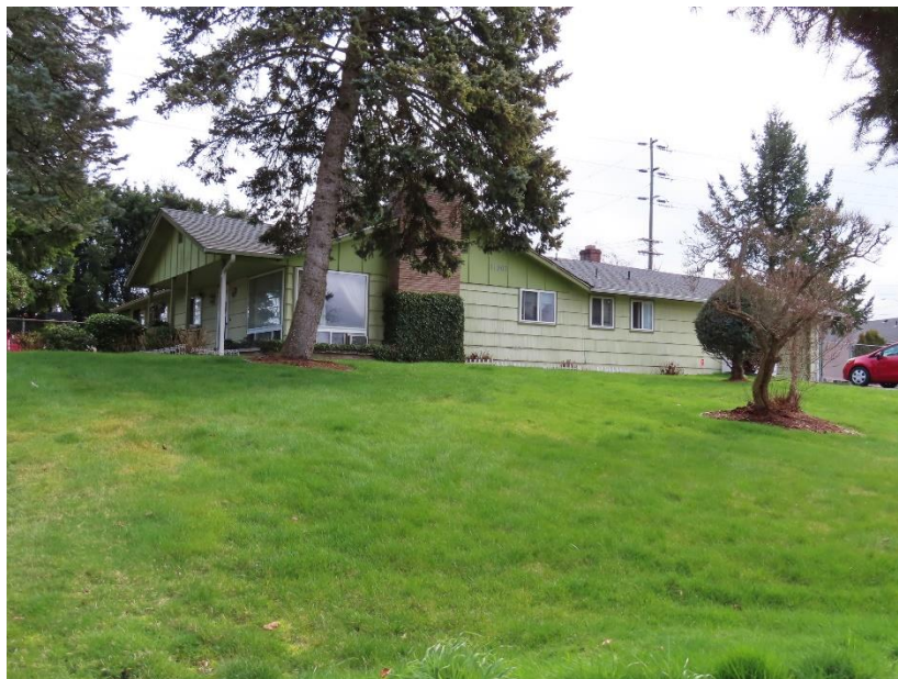
Figure 8-27 11803 Tomahawk Road SW, view southeast
