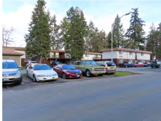
13020 Lincoln Avenue SW, view northeast.jpg
