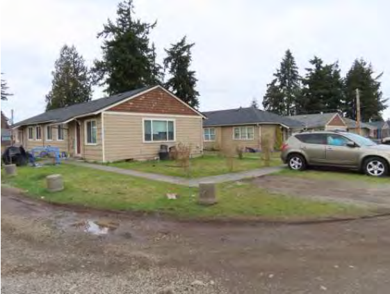
11216 through 11230 Kline Street SW, view
