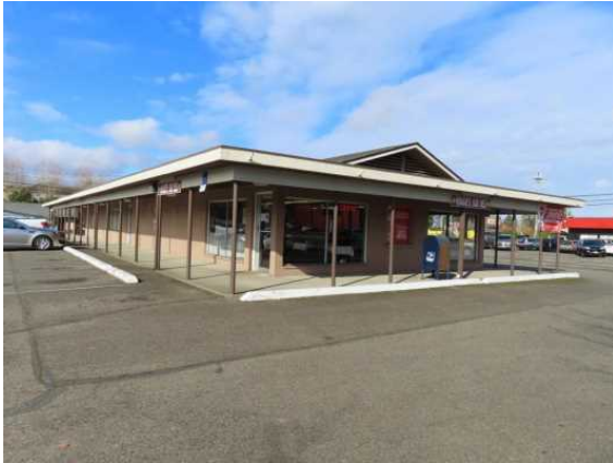
11202-11208 Bridgeport Way SW, view northwest..jpg
