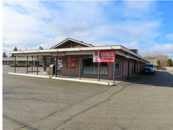
11202-11208 Bridgeport Way SW, view southwest.jpg
