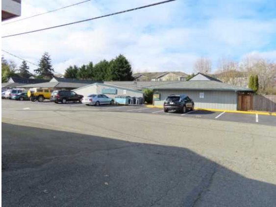
5202 112th Street SW, view southwest.jpg
