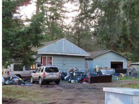
5508 Boston Avenue SW, view southwest.jpg
