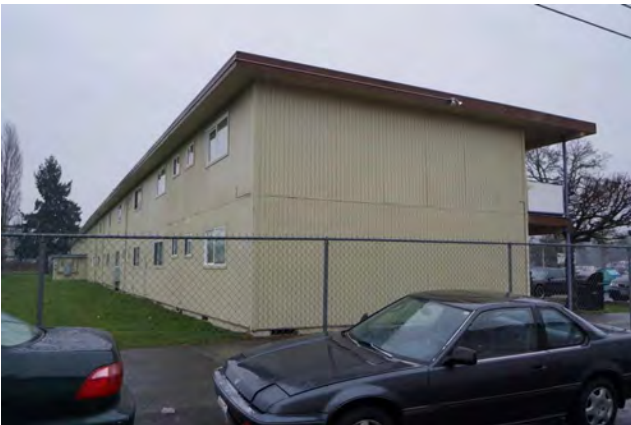
Northeast corner (back of building)
