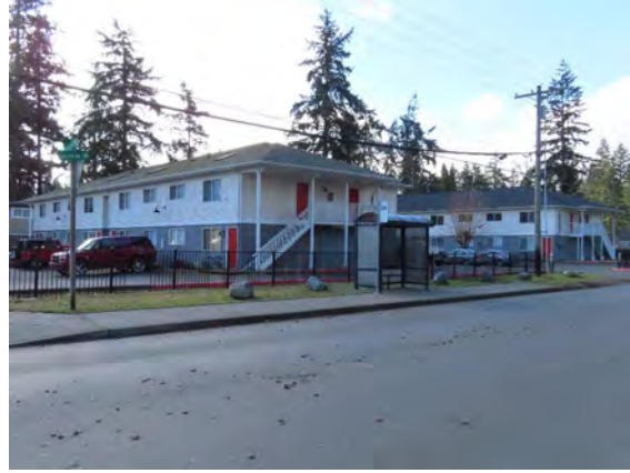
12809 Lincoln Avenue SW, view southwest.jpg
