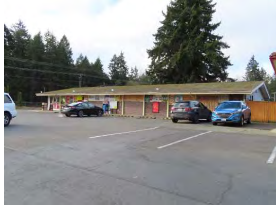
12928 Bridgeport Way SW, view southwest.
