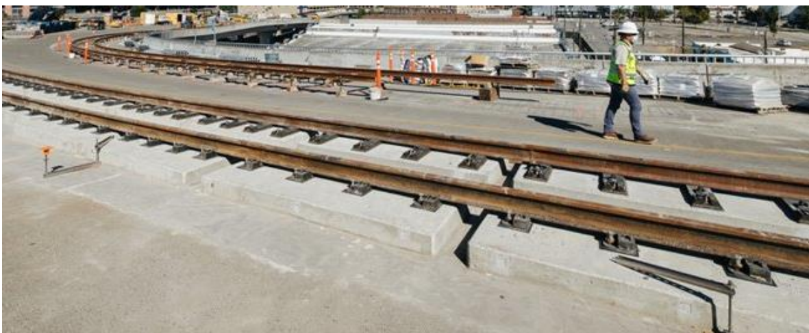
Fig. 2: Image showing concrete plinths supporting light rail tracks.
