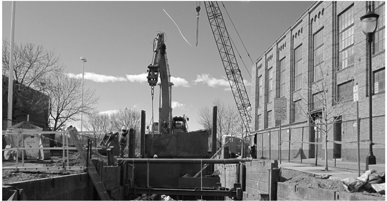
Dakota Outfall under construction from D4
