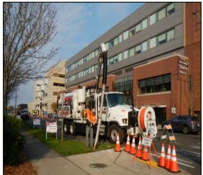
Picture Above: Utility potholing on MLK at MultiCare.
