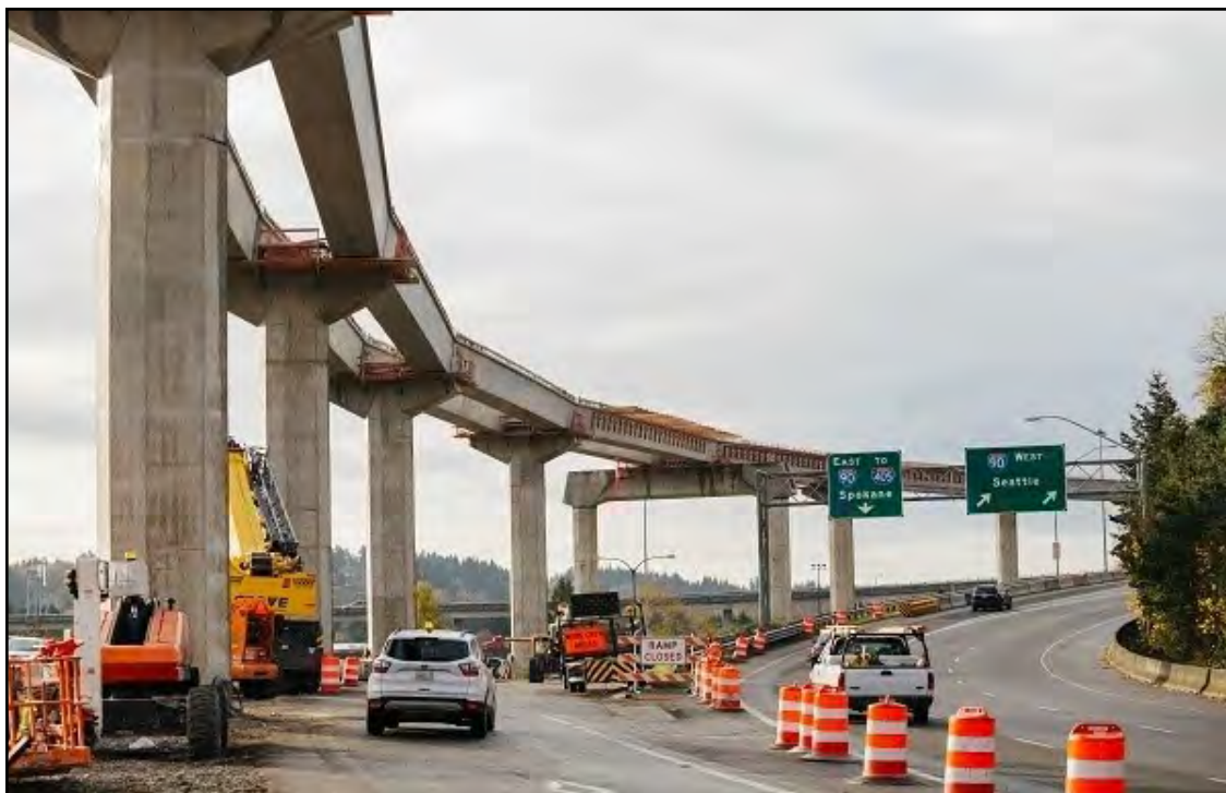
E320 South Bellevue: Columns and guideways leading to I-90.
