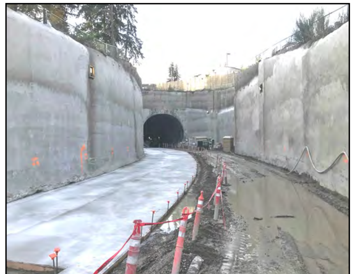
Mud slab poured on west half of South Portal cut-and-cover.
