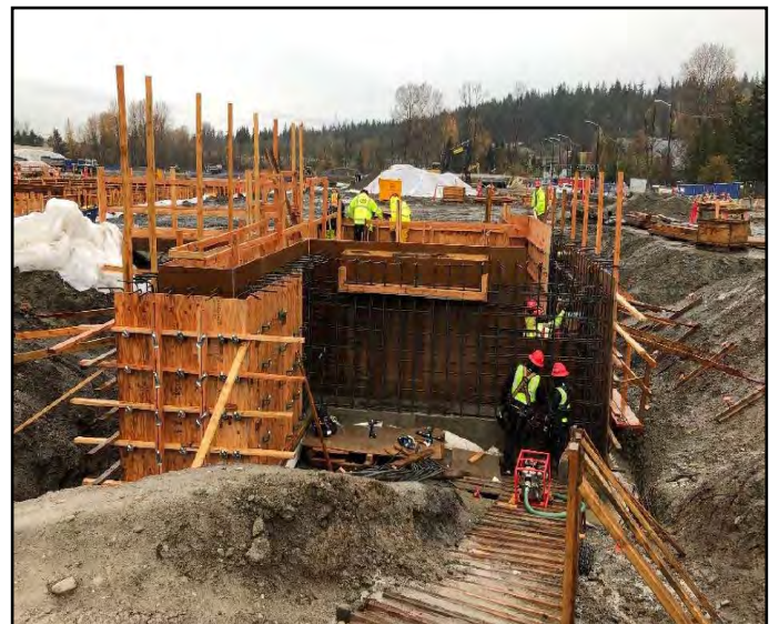
Wheel Truing Pit Rebar and Formwork.
