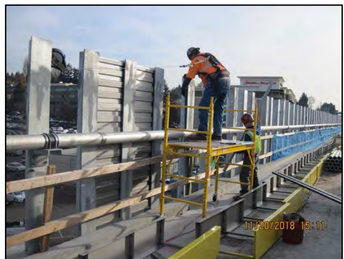
Installation of acoustical panels along Guideway.
