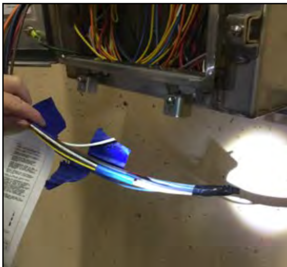
Checking wire terminations in tunnel control panels
