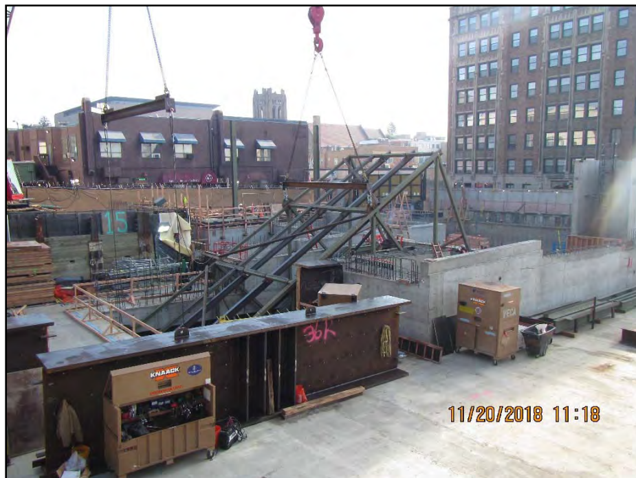
N140—South Circulation Tube Assembly Installation
