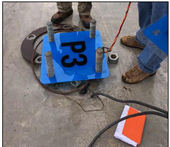
NG Station OCS Pole Foundation Verification, Nov 9, 2018.
