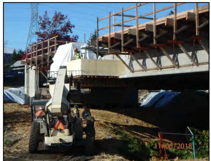
Installing OCS support forms on east bound span.
