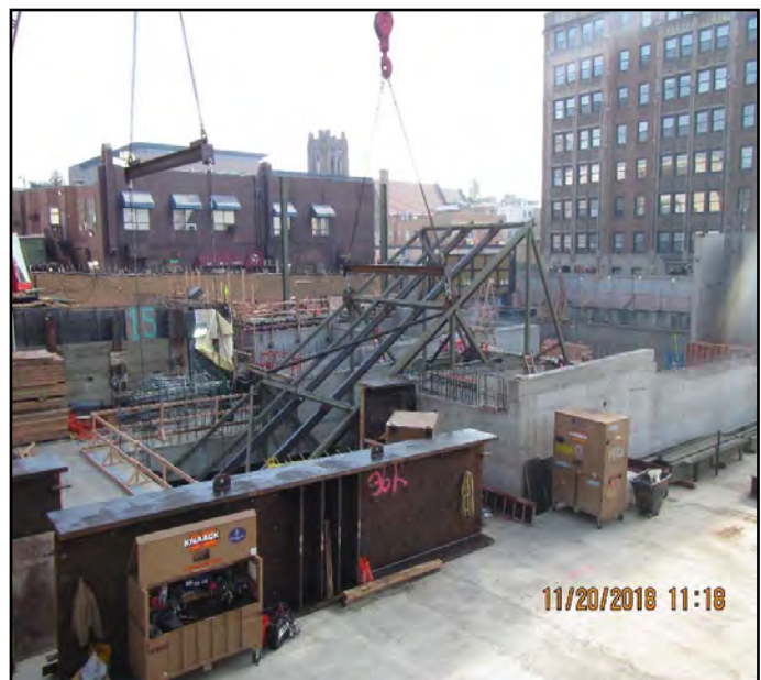
UDS – South Circulation Tube Assembly
