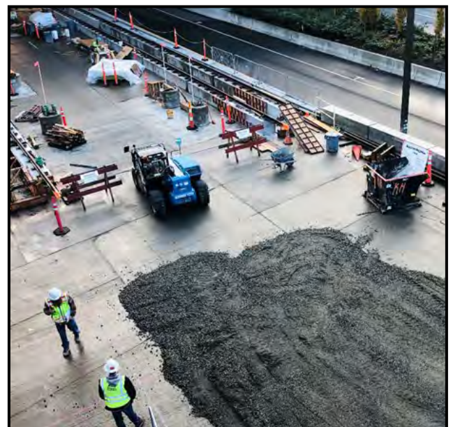
Sub-ballast placement, East Ballasted 1 transition area /MI Station
