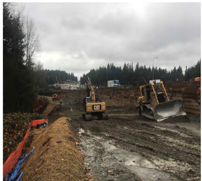
Grading temporary access road in Work Area 3.
