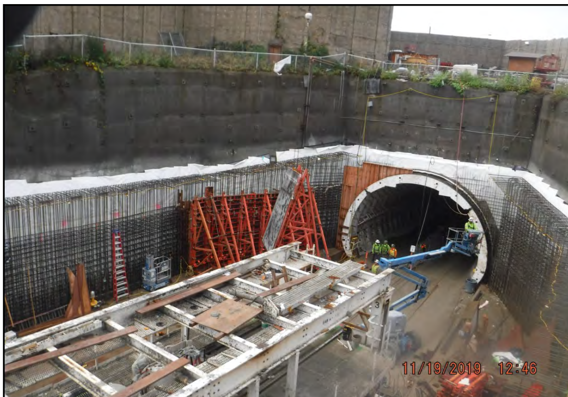
E330 Downtown Bellevue Tunnel: Rebar and formwork on south end of the tunnel portal.
