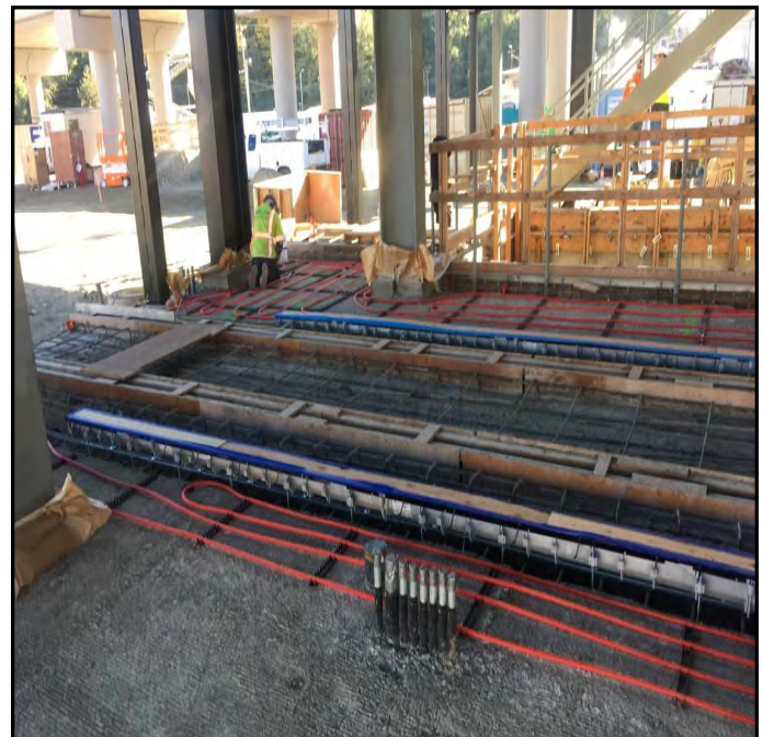
Floor Slab Preparation—OMF
