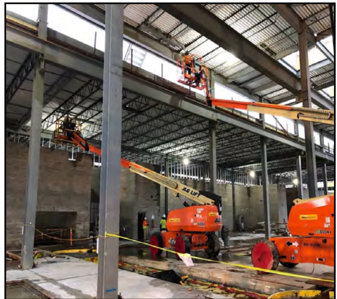
OMFE—Painting primer on unprimed steel members
