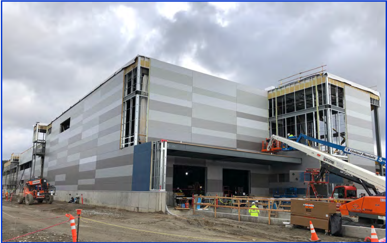
Exterior panel installation is ongoing at the OMF East
