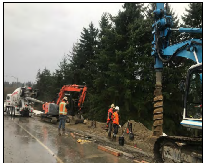
Drilling soldier piles for the SOE Walls in Work Area 1.
