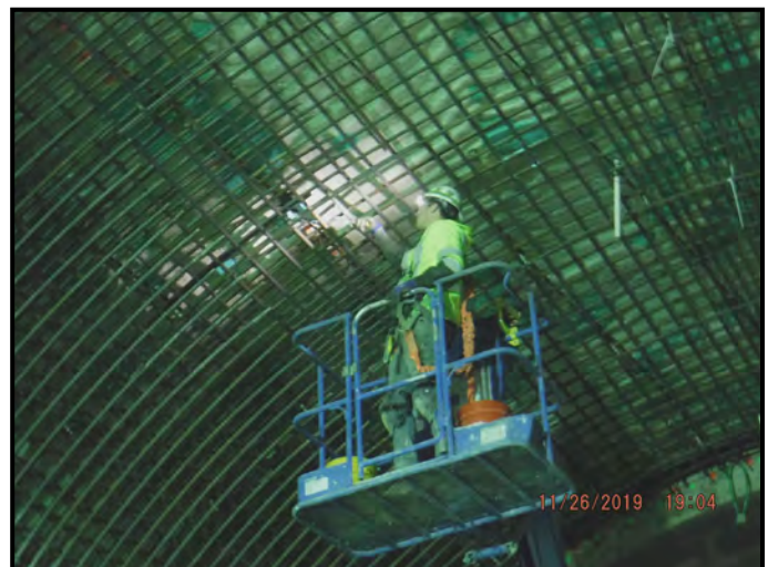
Waterproofing expanded zone crown.
