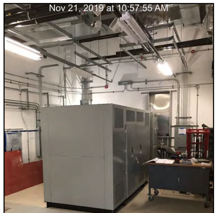
Setting TPSS Switchgear at UDS Station
