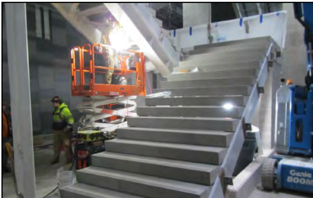
N140 – Precast Stair Treads on Added Stair 8.
