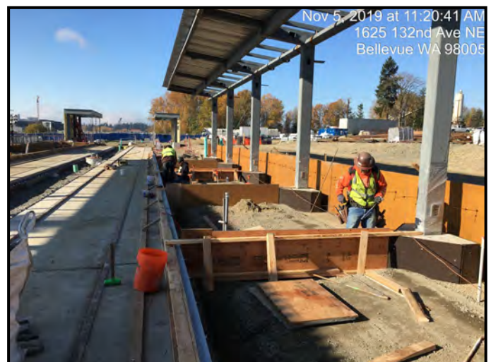
Forming the north-side station platform slab, looking north-west.
