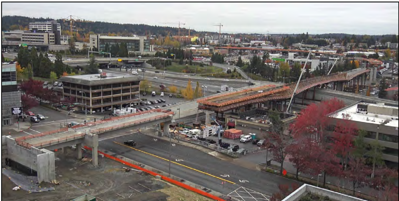
E335 Downtown Bellevue to Spring District: Bridging spanning over Highway I-405 along NE 6th Street
