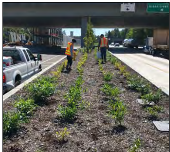
Plant Establishment review along I-90
