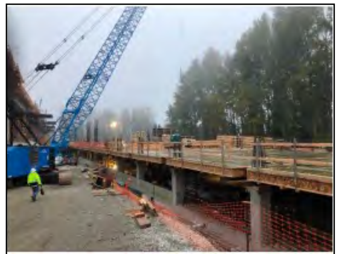
Parking garage work—second level
