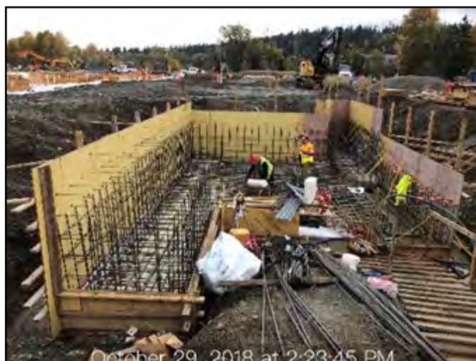
Wheel Truing pit rebar installation
