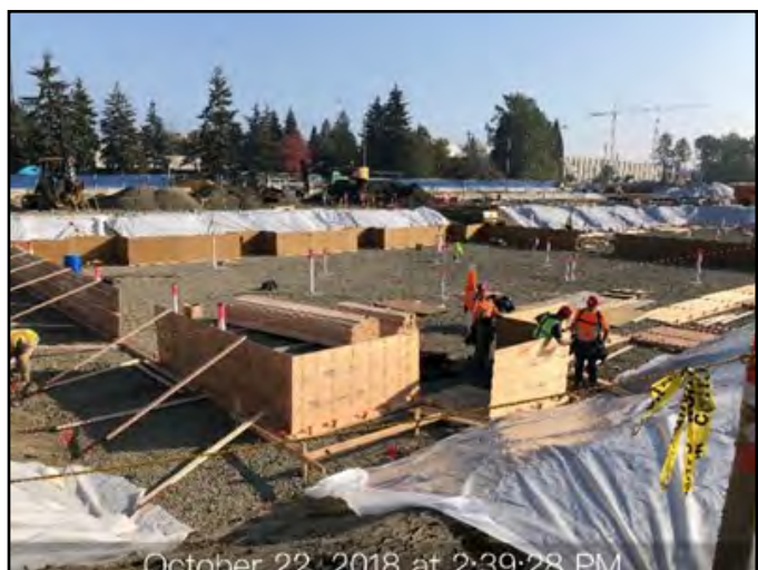
Forming LRV service Pit Area.
