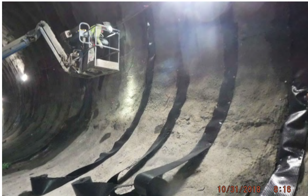
E330 Downtown Bellevue Tunnel: Installation of drainage mats in tunnel.
