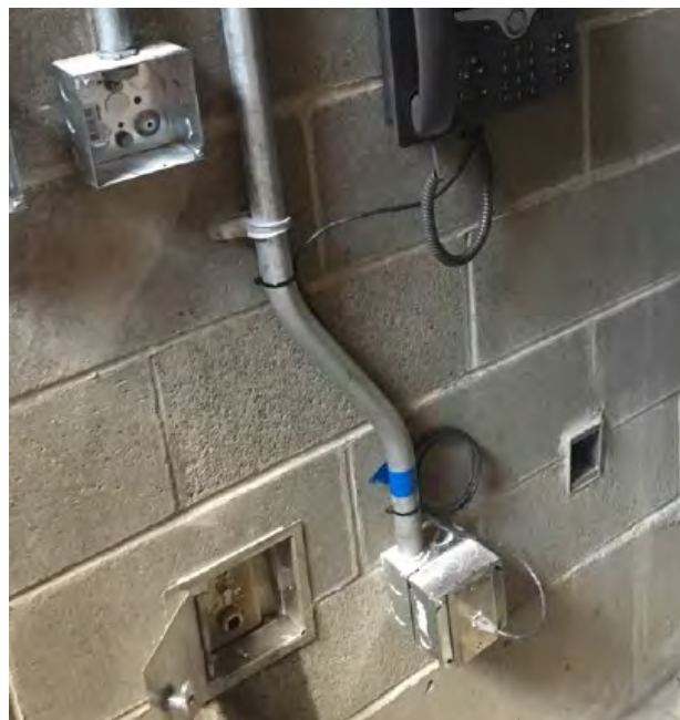
Punch list work at the Northgate Parking Garage.
