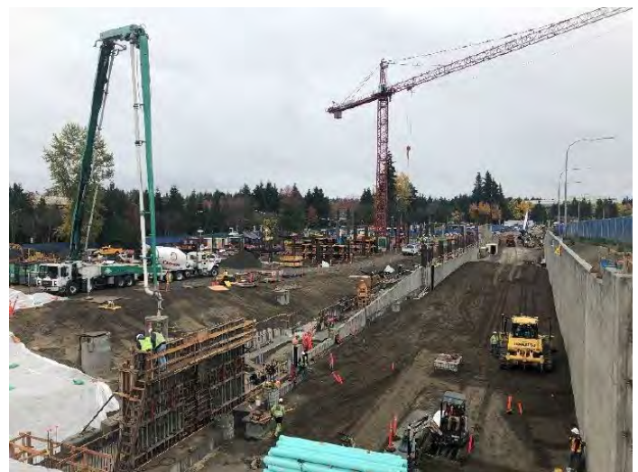
Redmond Technology Station Site Construction.
