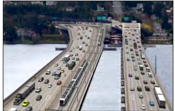
Since June 2017, the project has provided 24/7 HOV access on I-90 between Seattle, Mercer Island and Bellevue.
