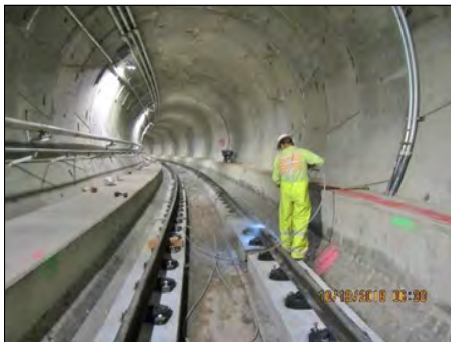
N180 — Crew cleaning debris off rail.
