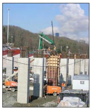
Figure 1-8 Falsework Columns Under Construction
