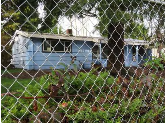
33531 18th Avenue S, view northwest.jpg
