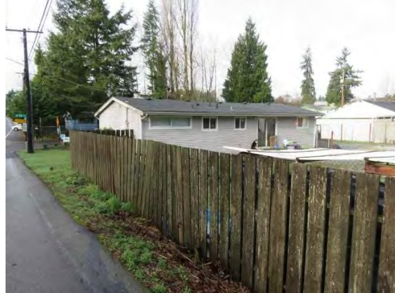
33532 18th Avenue S, view northwest.jpg
