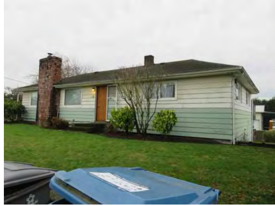
2907 S 244th Street, view southeast
