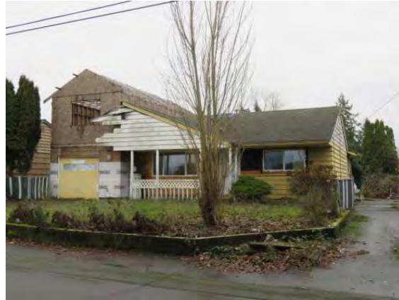
2911 S 252nd Street, view southeast.JPG
