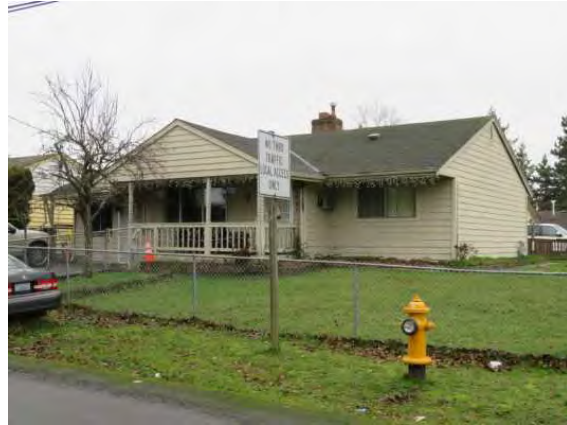
2905 S 252nd Street, view southeast.JPG
