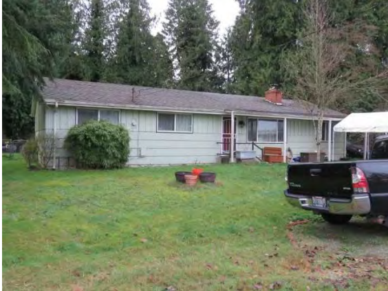
33025 24th Avenue S, view northwest.jpg
