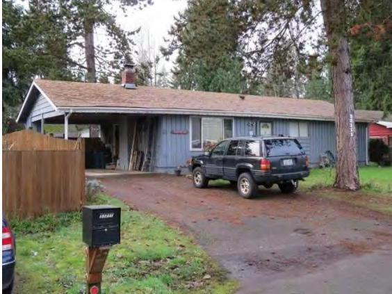
33111 24th Avenue S, view northwest.jpg
