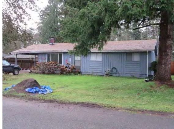
33111 24th Avenue S, view southwest.jpg
