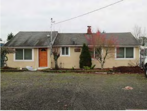
2859 S 244th Street, view south.JPG
