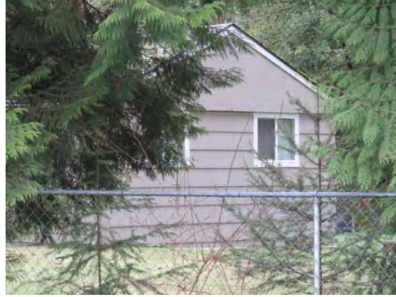
33003 24th Avenue S, view southwest.JPG
