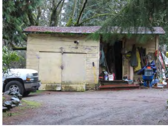
1828 S 340th Street outbuilding, view north
