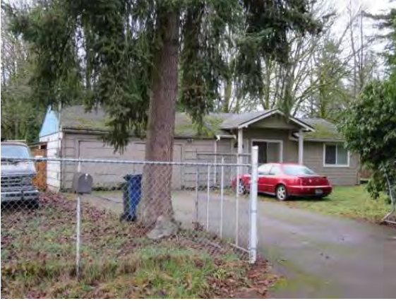
33003 24th Avenue S, view northwest.JPG
