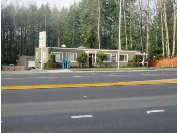
33903 Pacific Highway S, view northwest.jpg
