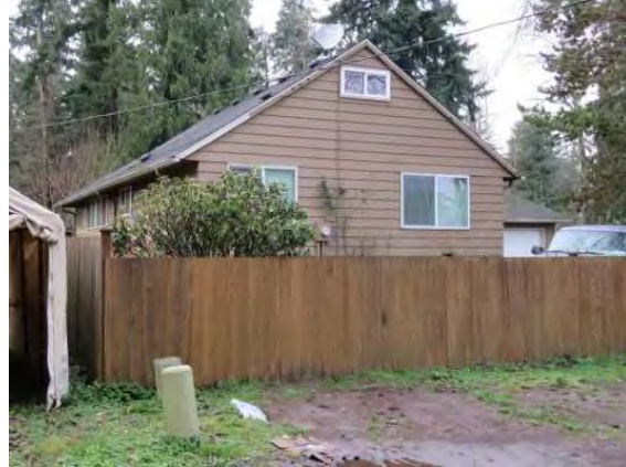
33211 24th Avenue S, view northwest.JPG
