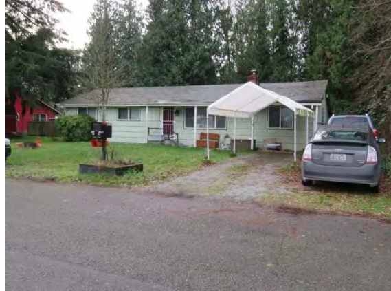
33025 24th Avenue S, view southwest.jpg
