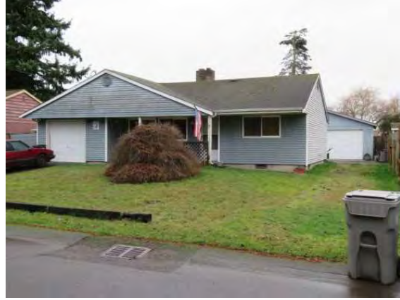
2933 S 252nd Street, view southeast.JPG
