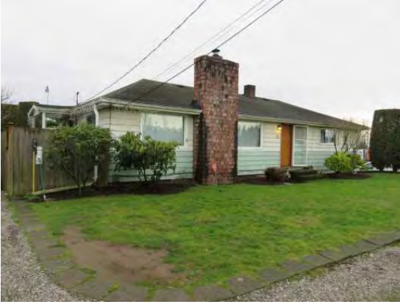
2907 S 244th Street, view southwest
