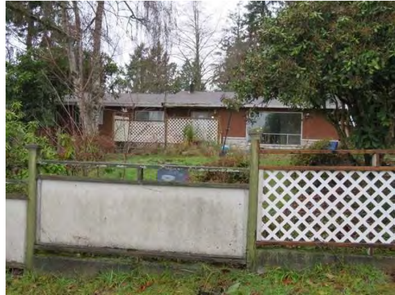
1724 S 340th Street, view north.jpg
