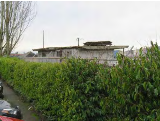
25036 Pacific Highway S, view northwest.JPG
