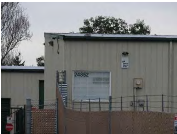
24852 Pacific Highway S, view east.JPG
