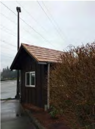
Northwest corner, entrance shed
