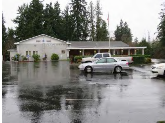
1700 S 340th Street, view north.jpg
