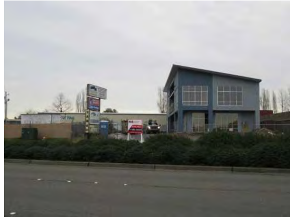
24852 Pacific Highway S, view east
