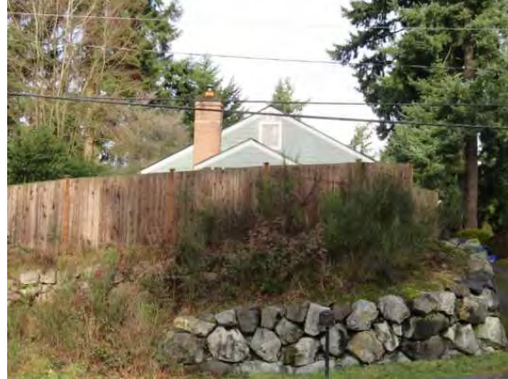
1820 S 336th Street, view north
