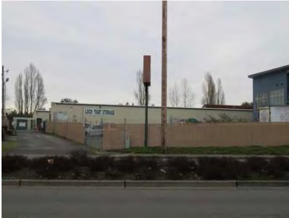
24852 Pacific Highway S, view southeast.JPG
