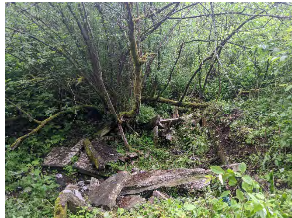
Figure G4.6-29 View of concrete basement with demolition debris, view east
