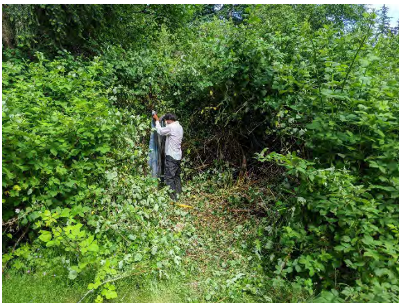
Figure G4.6-30 Cleared vegetation for excavation (SP01-17), view northeast
