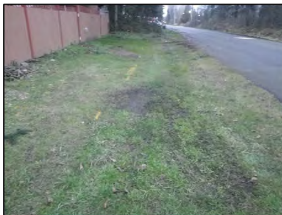
Figure G4.6-19 Marked buried natural gas pipeline (yellow paint) on the west side of 24th Avenue S, view north
