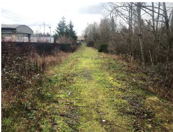
Figure G4.6-8 View of the levee along the western boundary of OMF 152, view north
