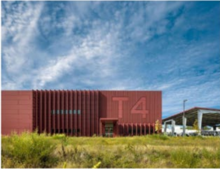
Applied large-scale elements
