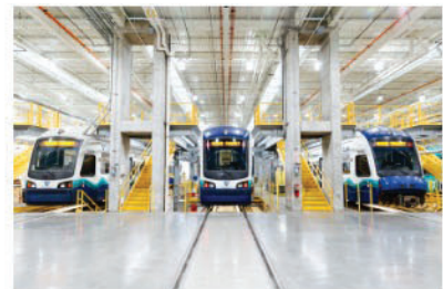
Link light rail cars receive nightly maintenance at the Seattle Operations and Maintenance Facility
