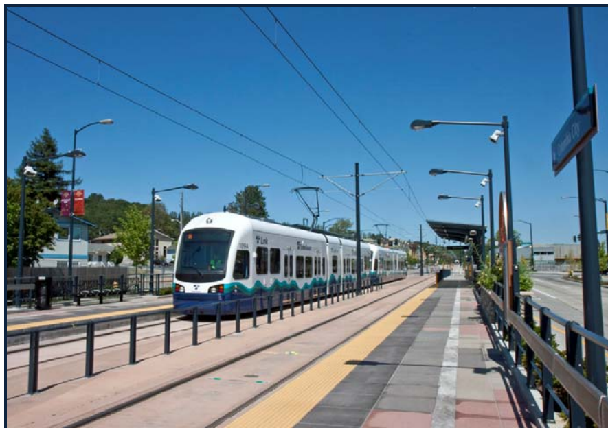
Central Link Light Rail Columbia City Station
