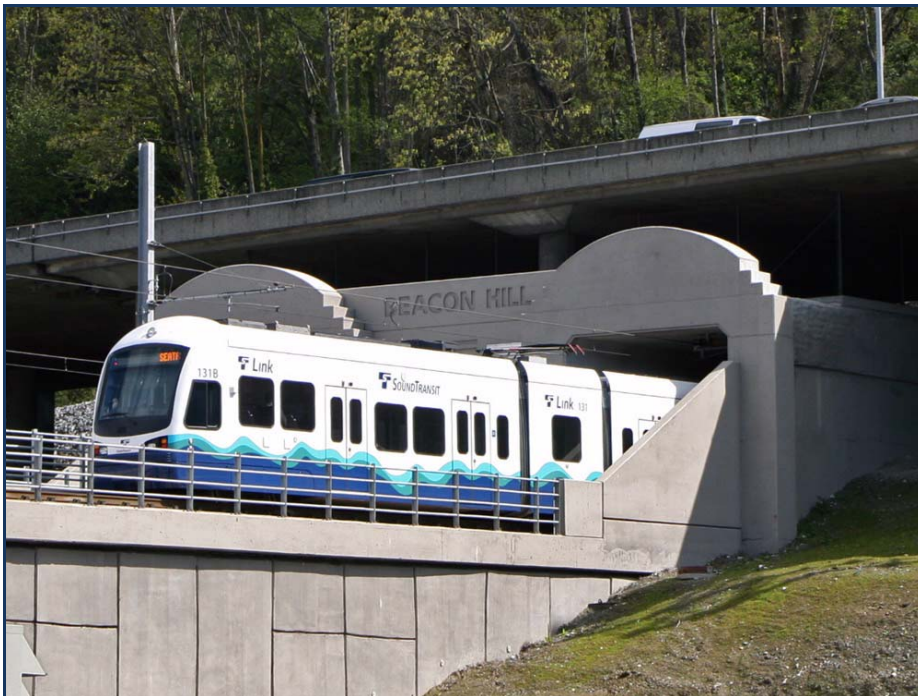
Central Link Light Rail Entering the Beacon Hill Tunnel
