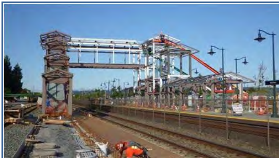
Construction of the Pedestrian Bridge Mukilteo Sounder Station – South Platform
