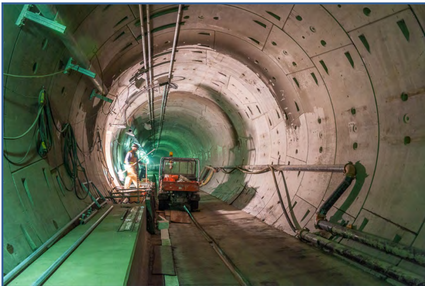
Tunnel Work for the Light Rail Extension from Seattle to the University of Washington
