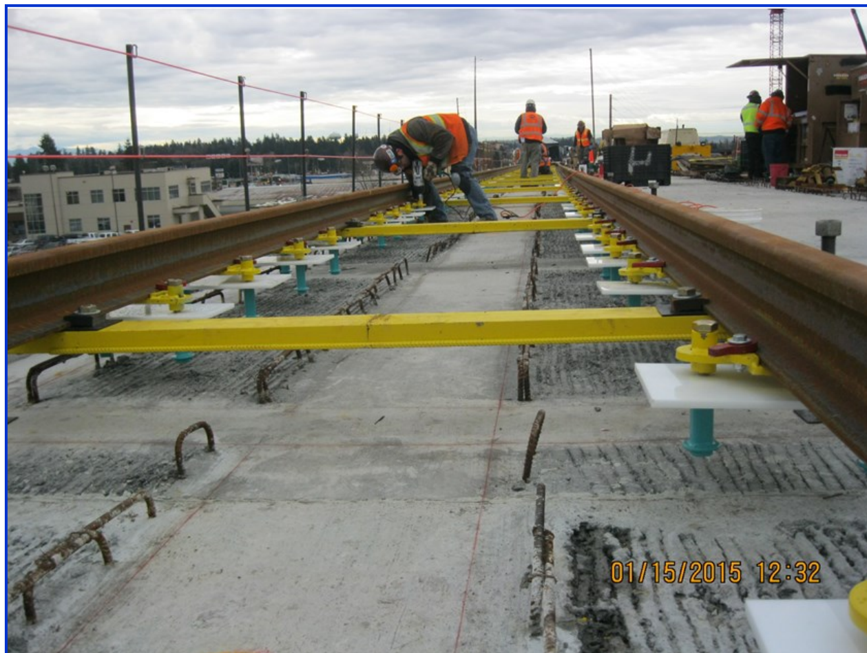
Preparation for track plinth pour for S. 200th Link Extension
