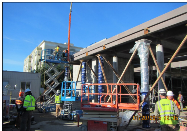
Concrete placement at West Entry of CHS.
