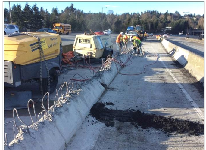
Demolishing existing concrete barrier on the I-90 East Channel Bridge as part of R8A Stage 3A HOV ramp construction.
