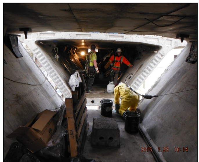
Gluing and scrubbing segments.
