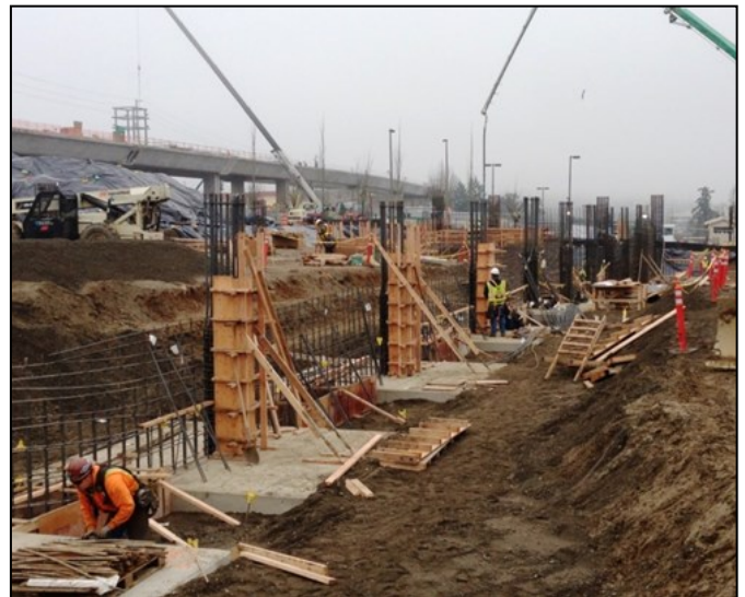
Workers installing forms and rebar for retaining wall.
