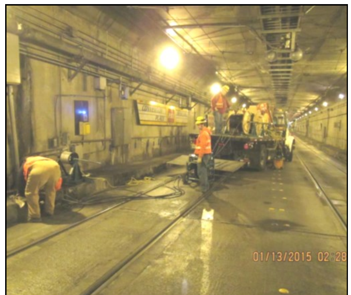
Signal system installation.
