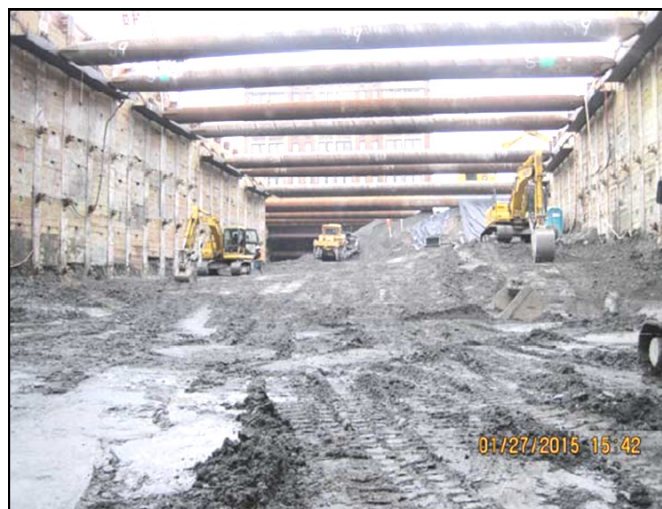
Excavating central shaft area at the U District Station shaft.
