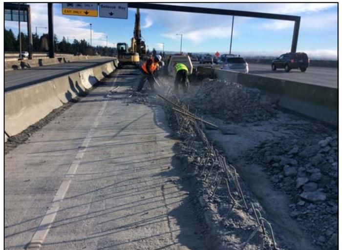
*Continued demolishing existing concrete barrier on I-90 for R8A Stage 3A HOV ramp construction.*
