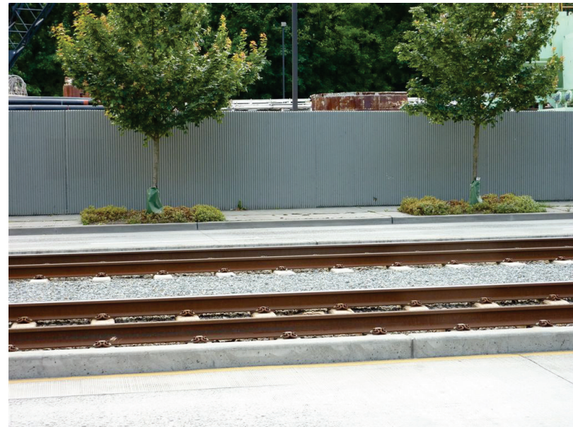
Figure 5. Example of at-grade sound wall
