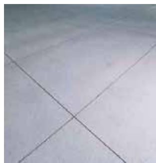
Concrete Pavement Proposed for station paving with sawcut scoring patterns. Two different score patterns will delineate the main circulation routes.
