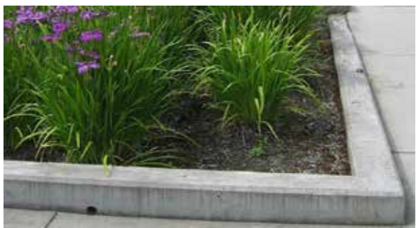
Bioretention Planters and areas proposed to receive rainwater collected from overhead platform and guideway and to receive stormwater runoff from surface parking areas.
