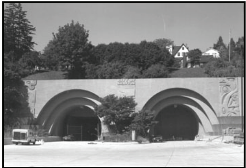
EXHIBIT 4.16-3 Mount Baker Ridge Tunnel
