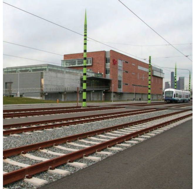
View of Sound Transit's Central Link Operations and Maintenance Facility in Seattle
