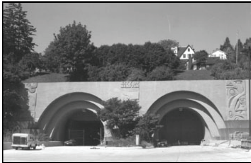
EXHIBIT 7-4 Mount Baker Ridge Tunnel
