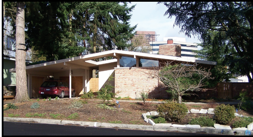
EXHIBIT 7-10 Mithun & Nesland Design at 11022 SE 2nd Street in Potential Surrey Downs Historic District
