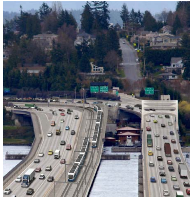
EXHIBIT 3-3 I-90 Floating Bridges with Visual Simulation of Light Rail in Center Roadway
