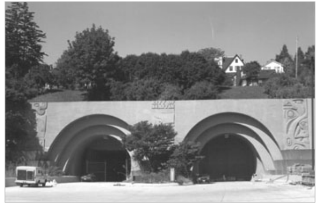
EXHIBIT 3-2 Mount Baker Ridge Tunnel, East End of I-90 Tunnel
