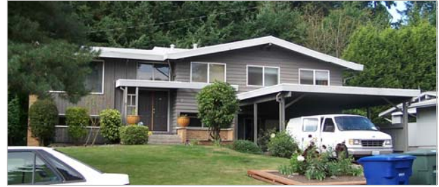
EXHIBIT 3-14 Split-Level Style at 301 109th Avenue SE
