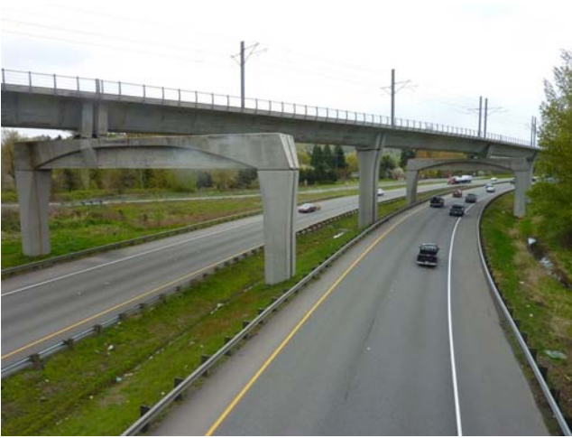
EXHIBIT D-24 Representative Straddle Bents Supporting a Light Rail Guideway
