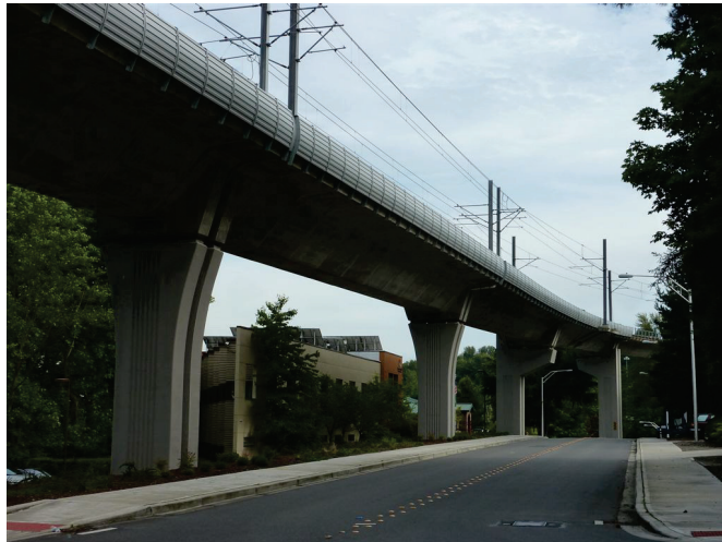
Figure 4. Example of sound wall on elevated structure
