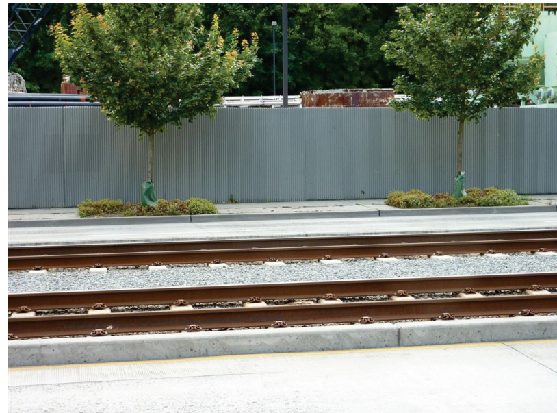
Figure 5. Example of at-grade sound wall
