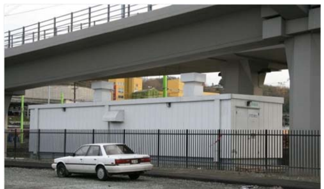
EXHIBIT 2-6 Traction Power Substation
