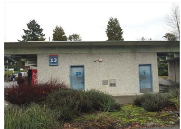
Highline College Building 13, West Elevation
