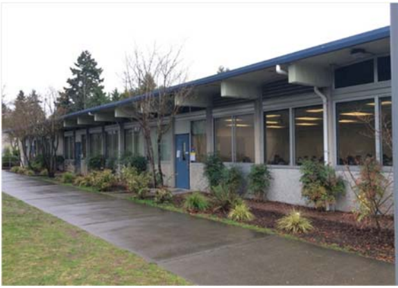
Highline College Building 14, North Elevation
