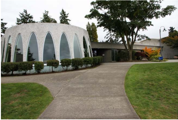
Highline College Building 4, West Elevation
