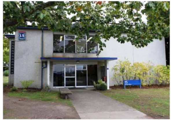
Highline College Building 15, West Elevation
