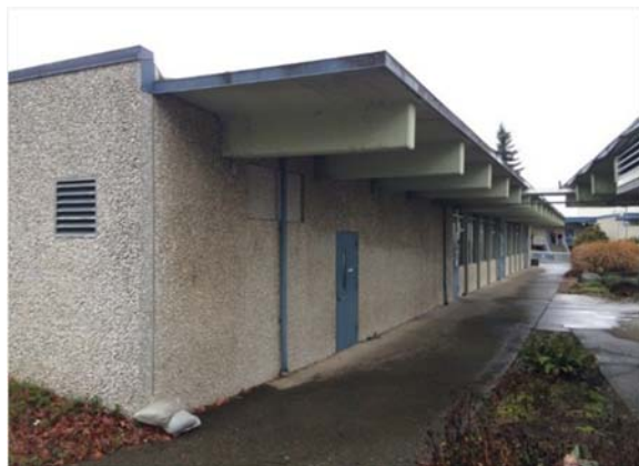
Highline College Building 12, Northeast Elevation
