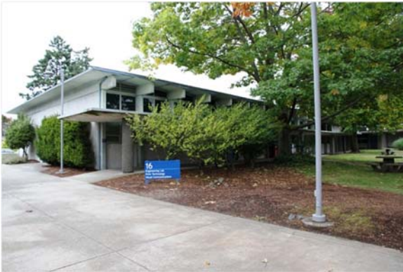
Highline College Building 16, Northeast Elevation
