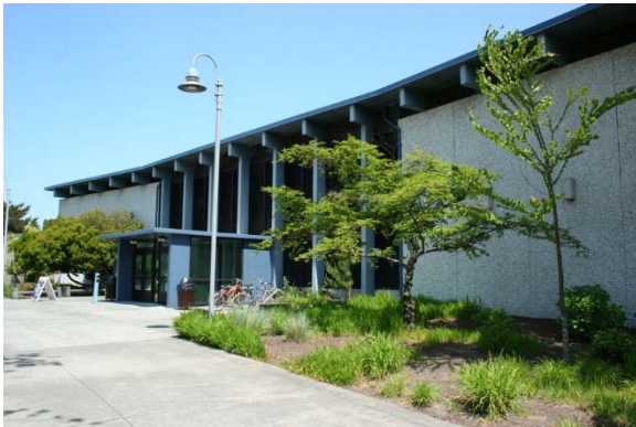
Highline College Building 6, West Elevation
