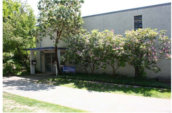
Highline College Building 5, Northwest Corner
