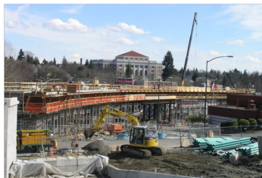
Staging Area Adjacent to the New Guideway Under Construction
