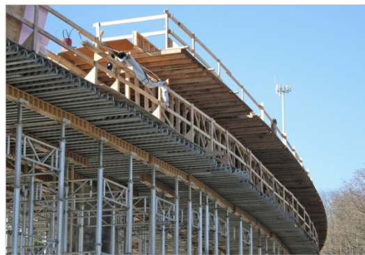
Construction of Elevated Guideway Showing False-Work
