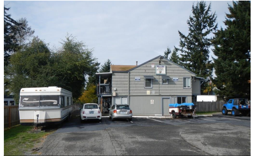
Photo 2: Looking west toward Lolani Apartments
