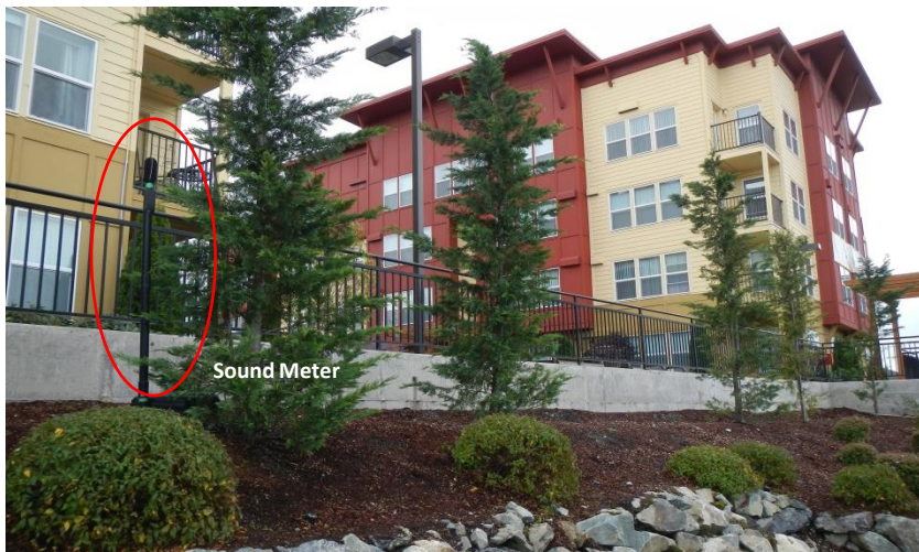
Photo 3: Looking southeast toward Viewpoint Apts.
