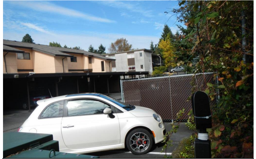
Photo 2: Looking northwest toward Access Condos
