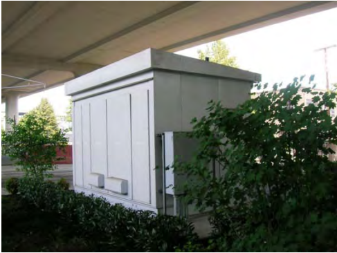
Figure 7 Typical Streetcar Traction Power Substation
