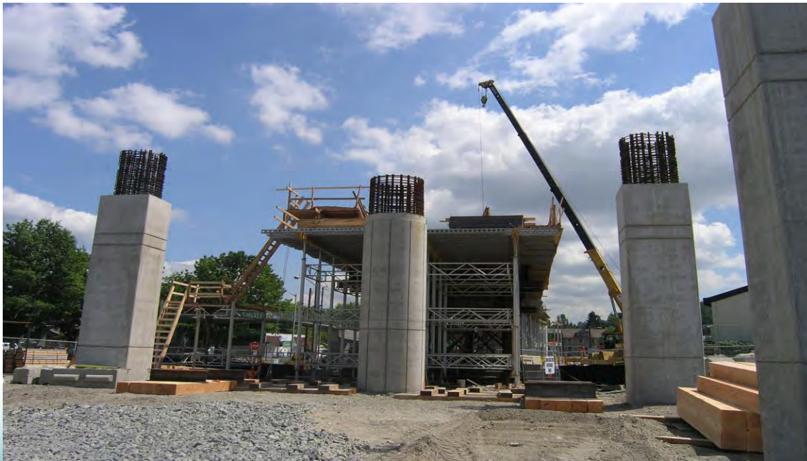
Mt Baker Station Station Construction
