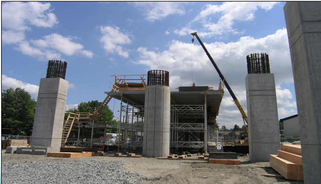
Mt Baker Station Station Construction
