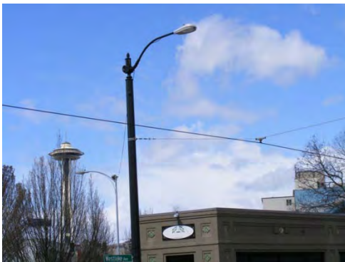
Figure 6 Single-wire OCS. Note span wire attachment to streetlight pole.
