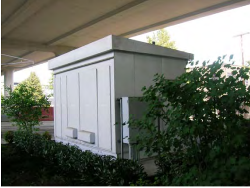
Figure 7 Typical Streetcar Traction Power Substation
