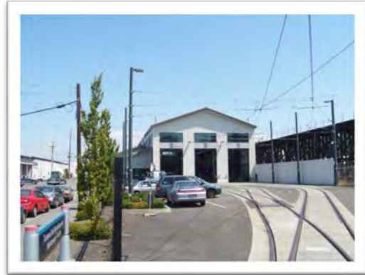
Figure 8 Existing Tacoma Link MSF
