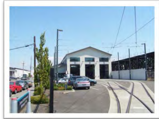
Figure 8 Existing Tacoma Link MSF
