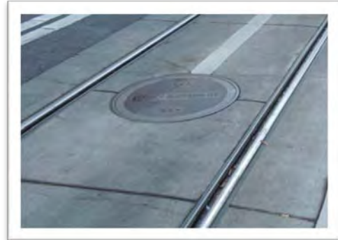
Figure 5 Shared use guideways provide better access to existing utilities than semi-exclusive guideways which guides utility accommodation policies.
